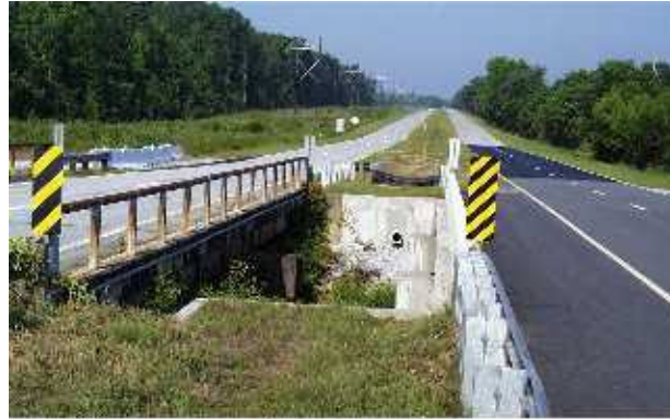
Figure 3 - Bridges 71G and 72G
