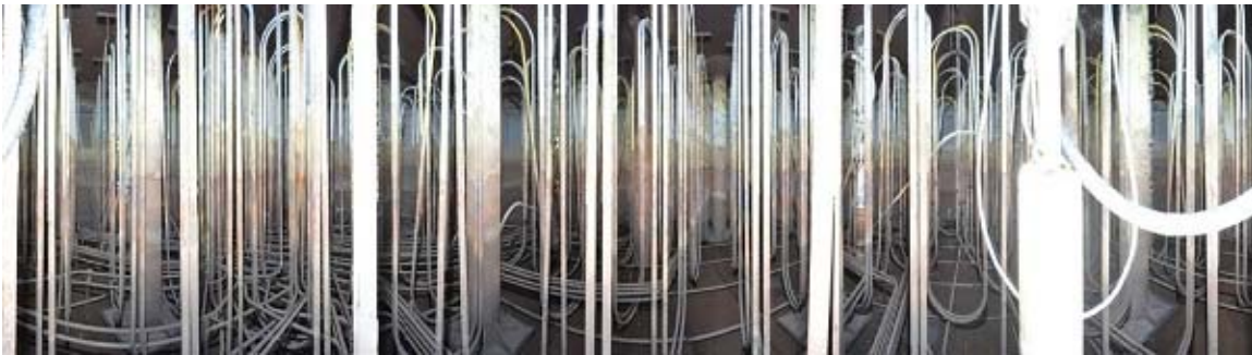
Fig. 5: High Resolution Photographs of Tank Interior
