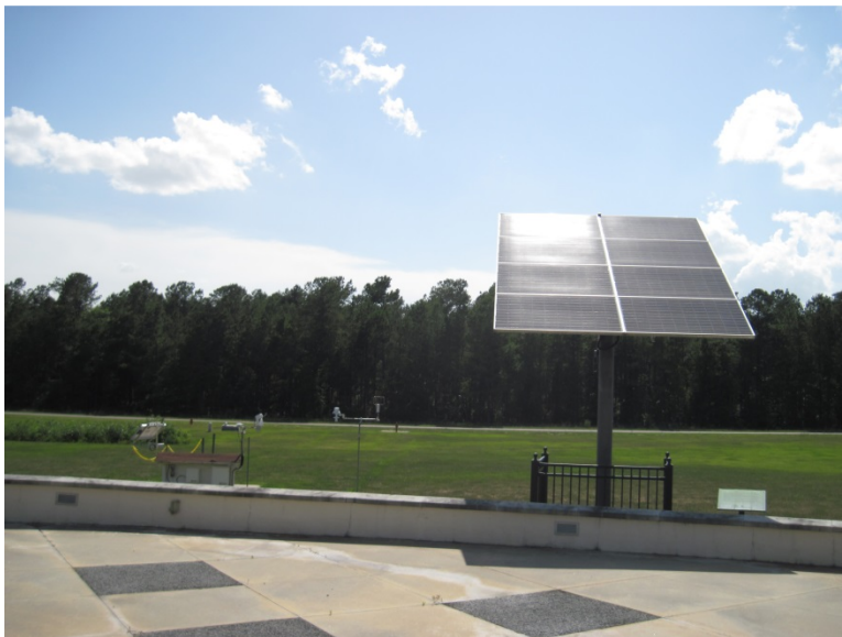
Solar monitoring station radiometer installed at the ARC.
