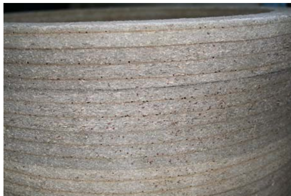
Drugstore Beetle Bore Holes in Celotex™ Lower Subassembly
