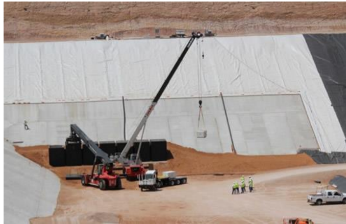
Figure D-5. Wastes Being Loaded into Modular Concrete Canisters at the Waste Control Specialists Disposal Cell
