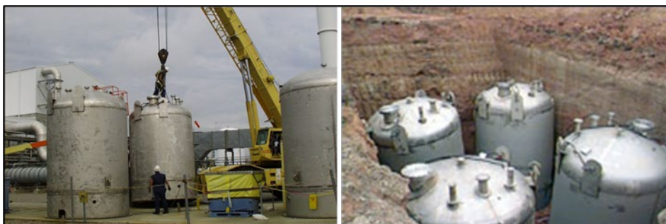
Figure 4-59. ETF Activated Carbon Columns Being Prepared for Shipment to E-Area (left) and Disposed in ST03 (right)
