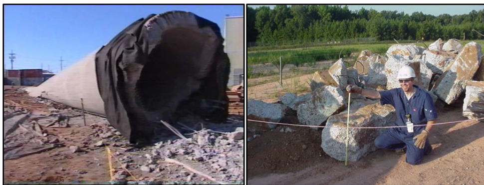
Figure 4-66. Concrete Rubble from 232-F Demolition Activities: Dropping of the 232-F Concrete Stack (left) and Resulting Concrete Rubble (right)
