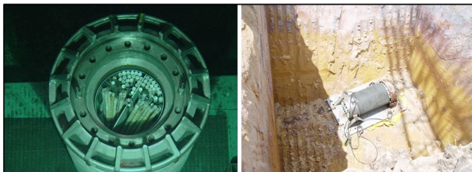
Figure 4-61. Paducah Demonstration Cask Loaded in L-Area at Savannah River Site (left); Sealed Cask Placed in ST05 on May 27, 2004 (right)
