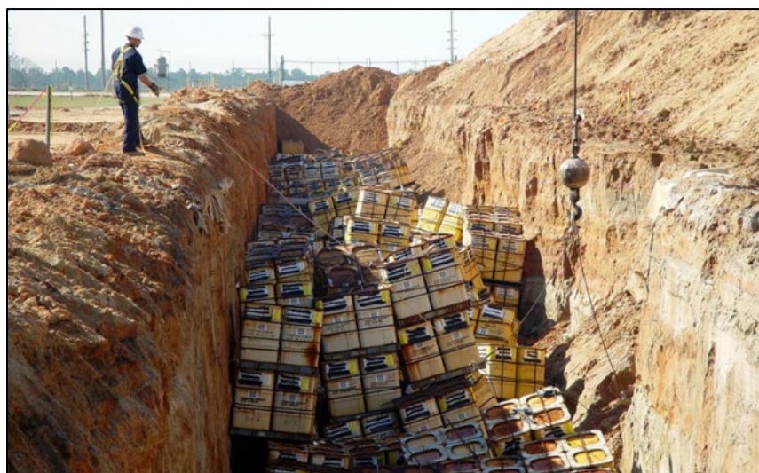
Figure 4-60. Disposal of Containers of Vitrified M-Area Glass in ST02 in 2003
