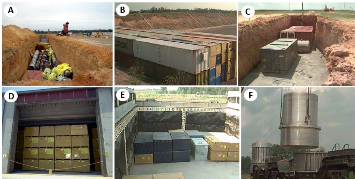
Figure 1-3. Operational Photographs of E-Area Low-Level Waste Facility Units: A) Slit Trench; B) Engineered Trench; C) Components-in-Grout Trench Segment; D) Low-Activity Waste Vault; E) Intermediate-Level Vault; F) Naval Reactor Component Disposal Area
