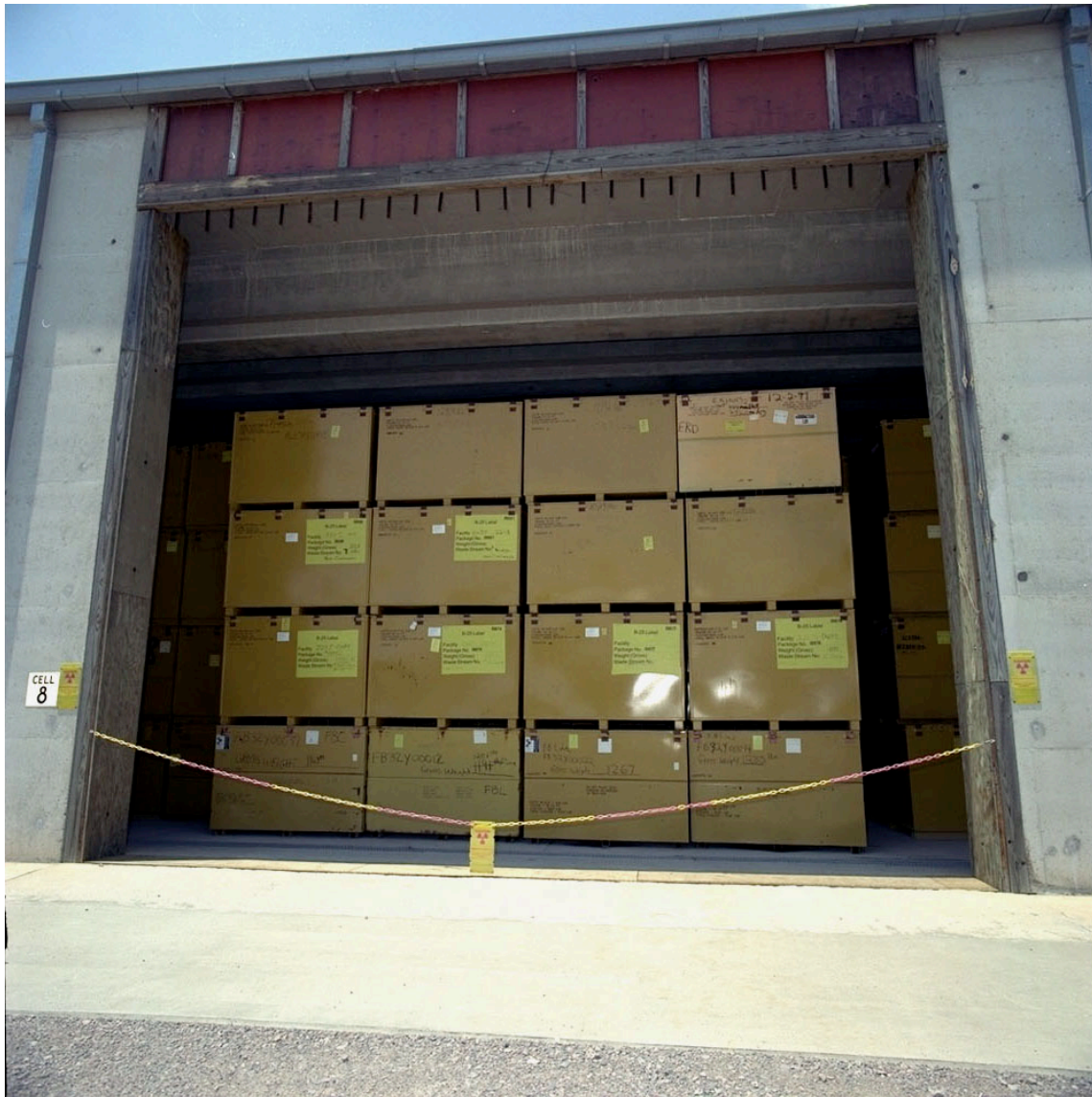
Figure 2-2 Interior View of LAWV Cell.
