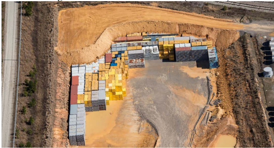
Engineered Trench #3 View from Berm (3-15-2016)
