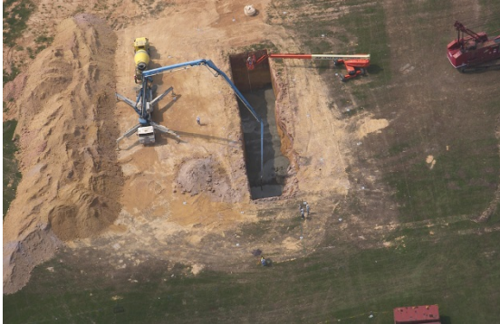
Emplacement of Bottom Foot of Grout
