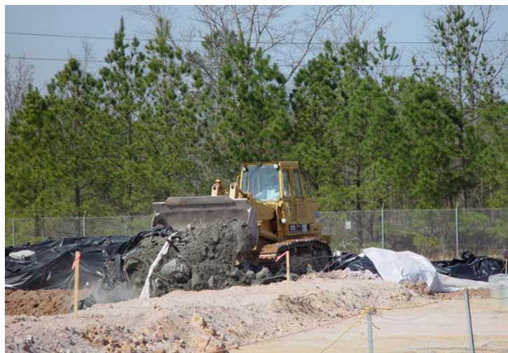
Figure 4-10. Operational Slit Trench Photographs
