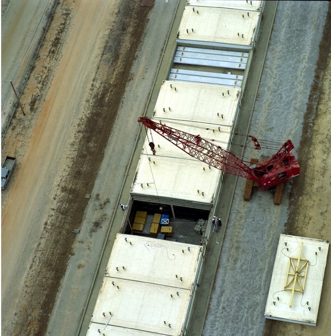
Figure 4-17. IL Vault aerial view
