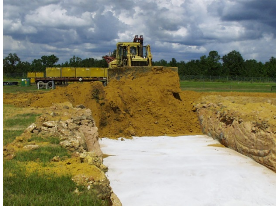
4-Foot of Clean Soil Cover
