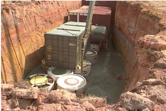
Grouting Sides of Segment
