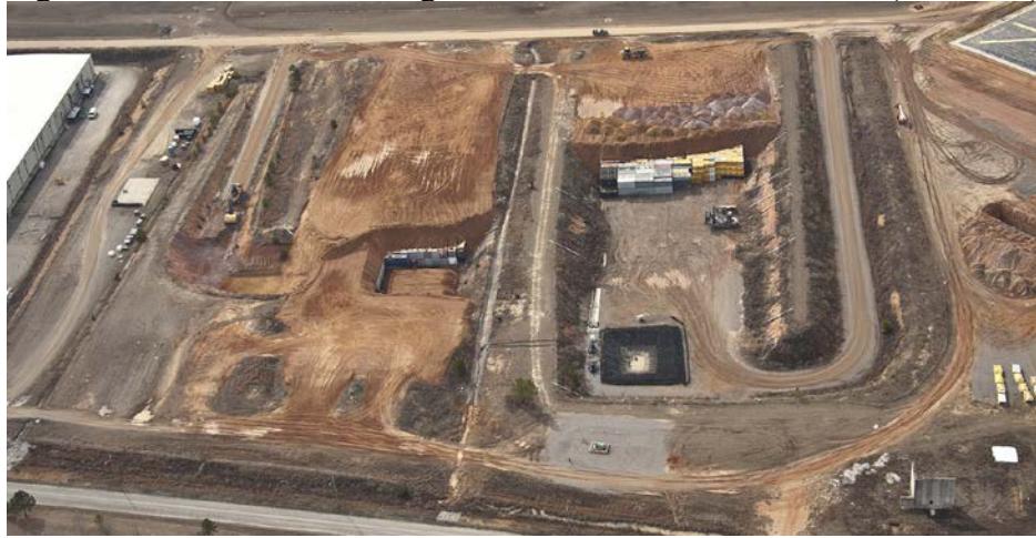
Engineered Trench #1 and Engineered Trench #2 Aerial View (2-2-2011)
