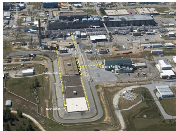
Fig. 1 - H-Canyon Facility with tunnel locations noted
