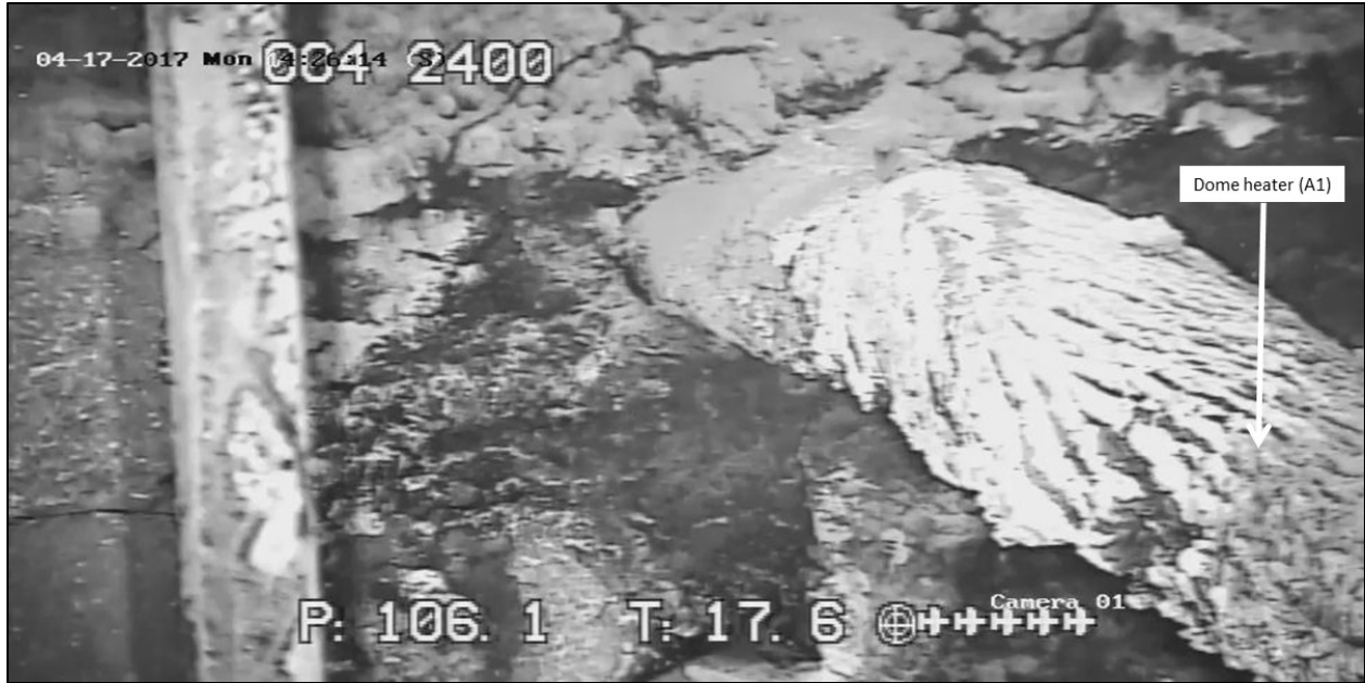
Figure 5-11. Dome heater penetrations, upper pair (A), northeast side of melter
