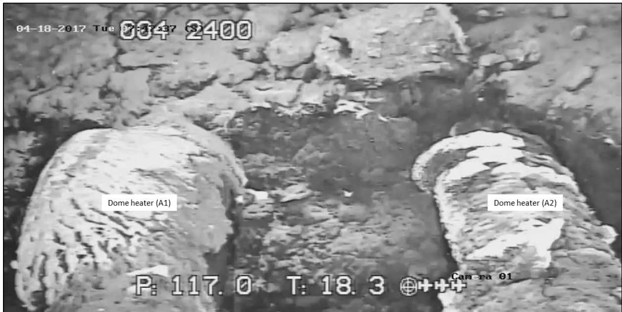
Figure 5-12. Dome heater penetrations, upper pair (A), northeast side of melter, alternate view
