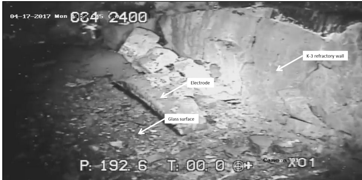
Figure 5-22. Upper electrode, southeast side of melter
