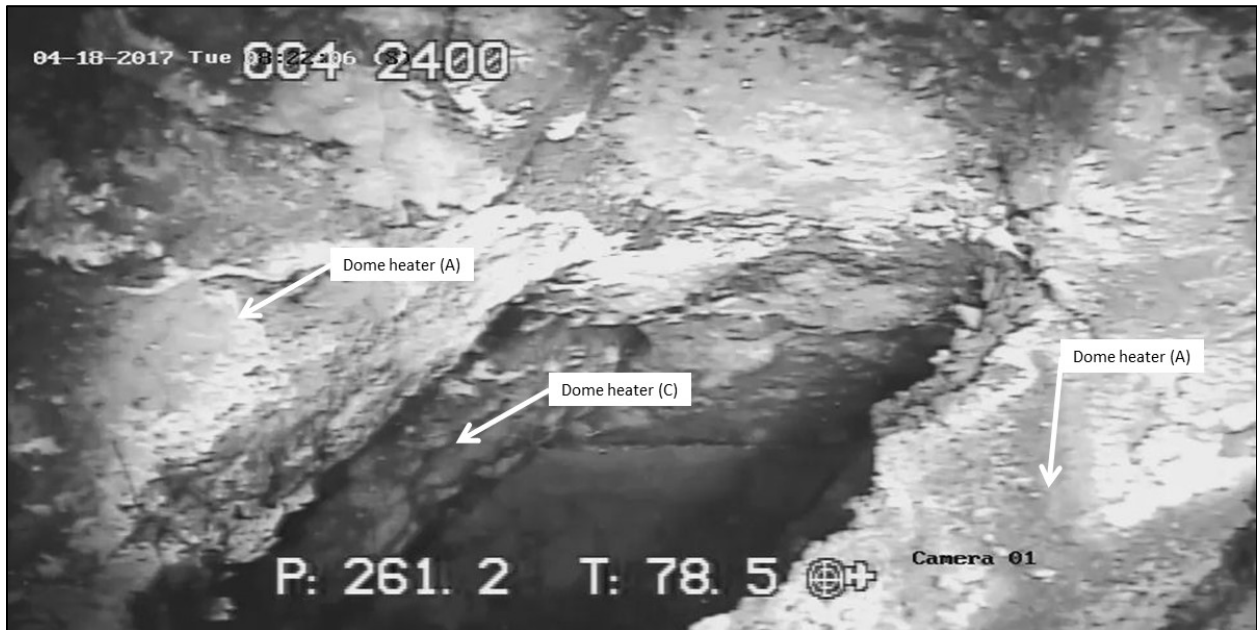
Figure 5-16. Dome heater penetrations, southeast side of melter, view from above
