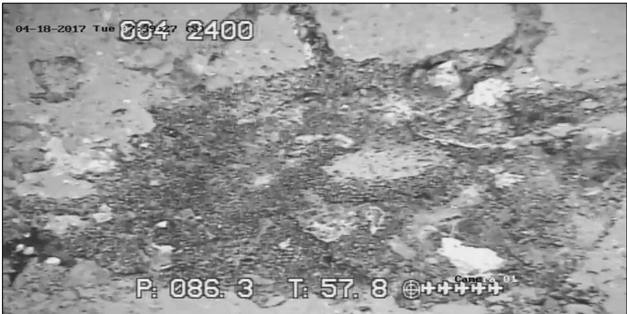
Figure 5-41. Closer view of cracked material atop mound
