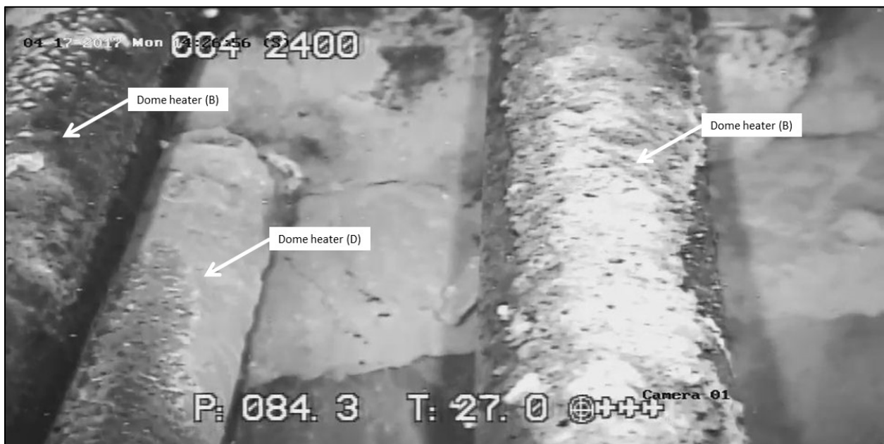
Figure 5-9. Deposits on dome heaters
