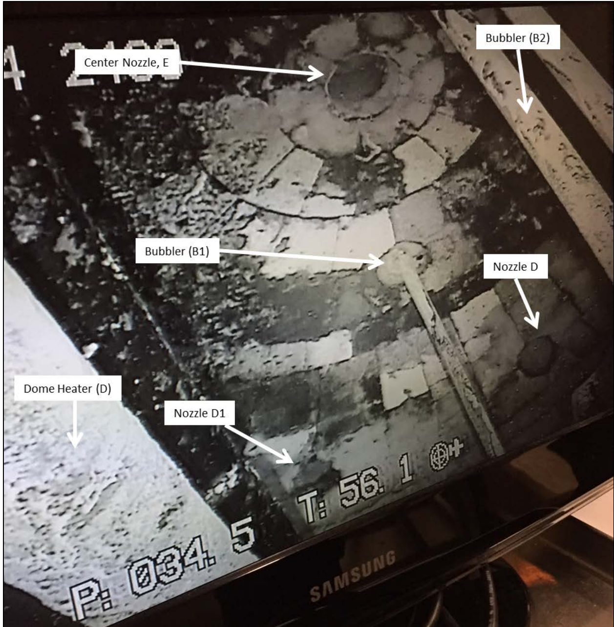
Figure 5-5. Underside of Melter 2 top head showing vapor space refractory and nozzle penetrations
