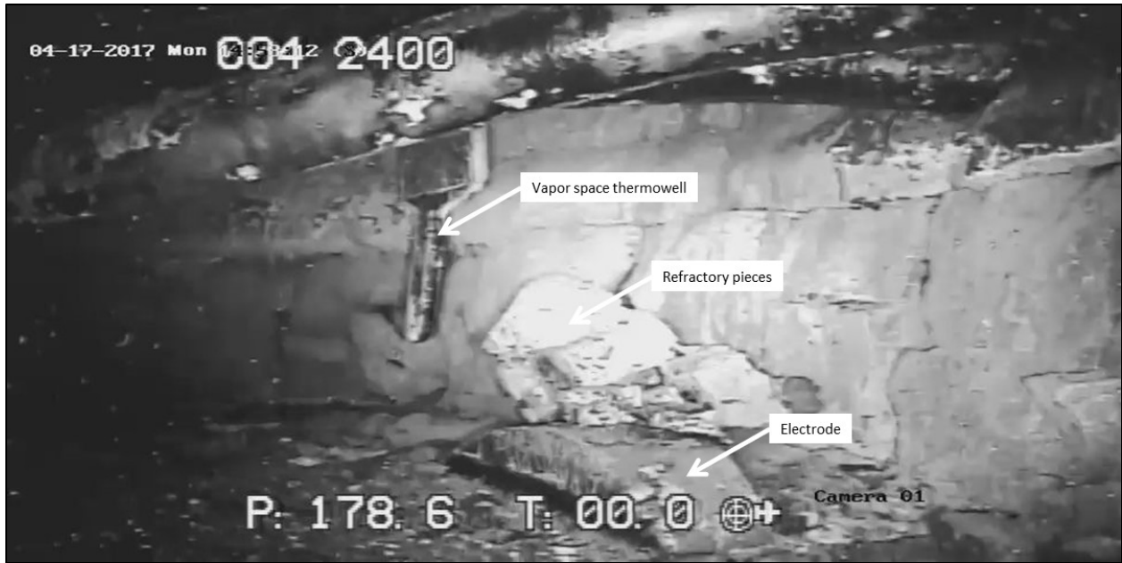
Figure 5-23. Refractory pieces visible behind upper electrode
