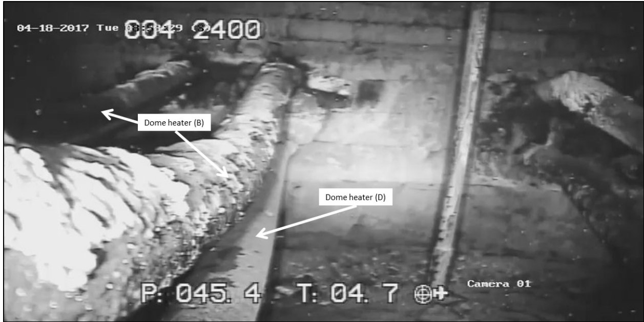
Figure 5-20. View along dome heaters showing deformation, west side of melter
