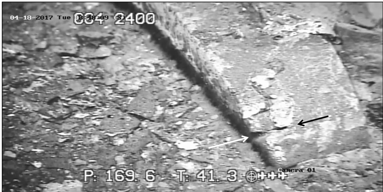
Figure 5-28. Larger crack visible on top of upper electrode, southeast side of melter
