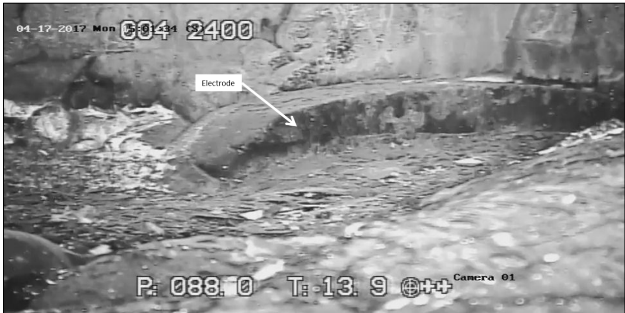
Figure 5-30. Detail view of upper electrode (L3), northwest side of melter
