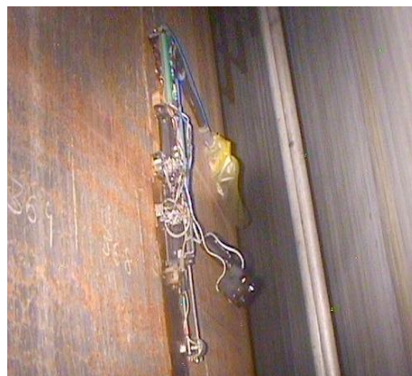
Figure 5a: In-use UT Wall Crawler with P-Scan Device.
