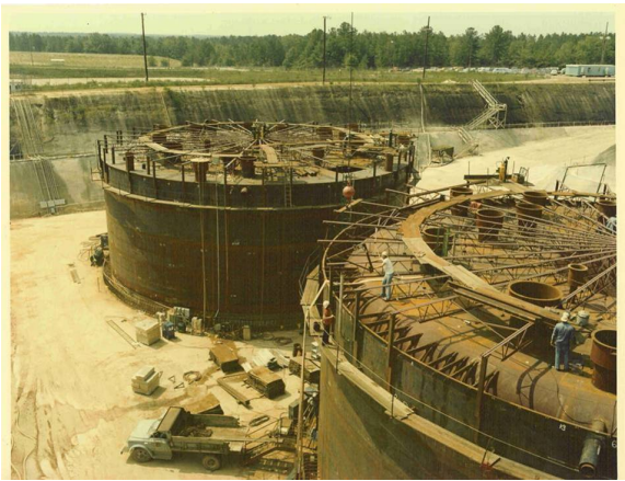
Figure 1: Type III LW Tank under Construction during the 1960s.
