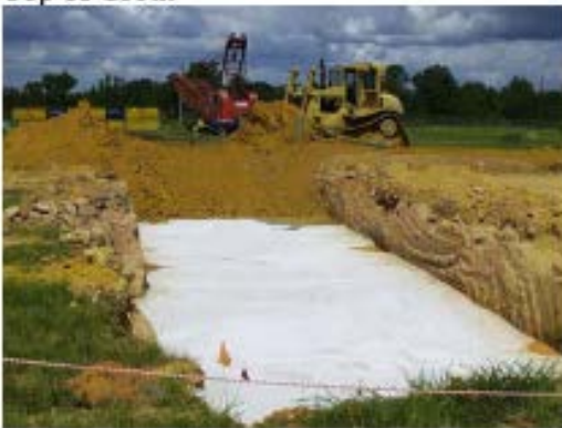
Top of Grout
