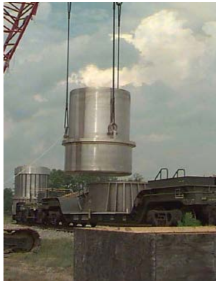
Figure 15. (Top) Photo showing partially covered naval reactor components of various sizes. Earth and a clay cap will be mounded over naval reactor waste prior to final closure. There are two such facilities, the “old” (two top photos) and “new” (bottom photo) facilities. (Bottom) Naval reactor component before it is placed in the disposal area (WSRC 2008).
