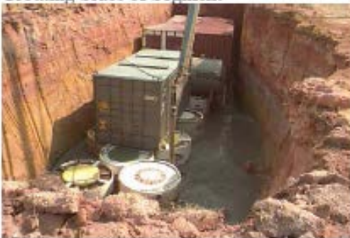
Grouting Sides of Segment
