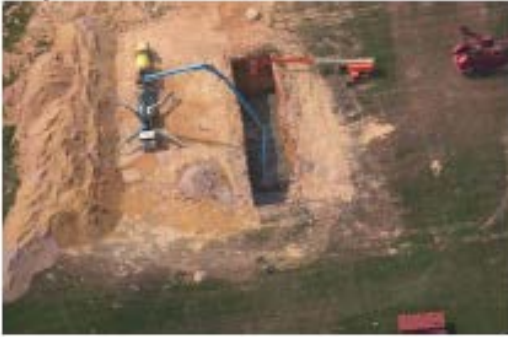
Emplacement of Bottom Foot of Grout
