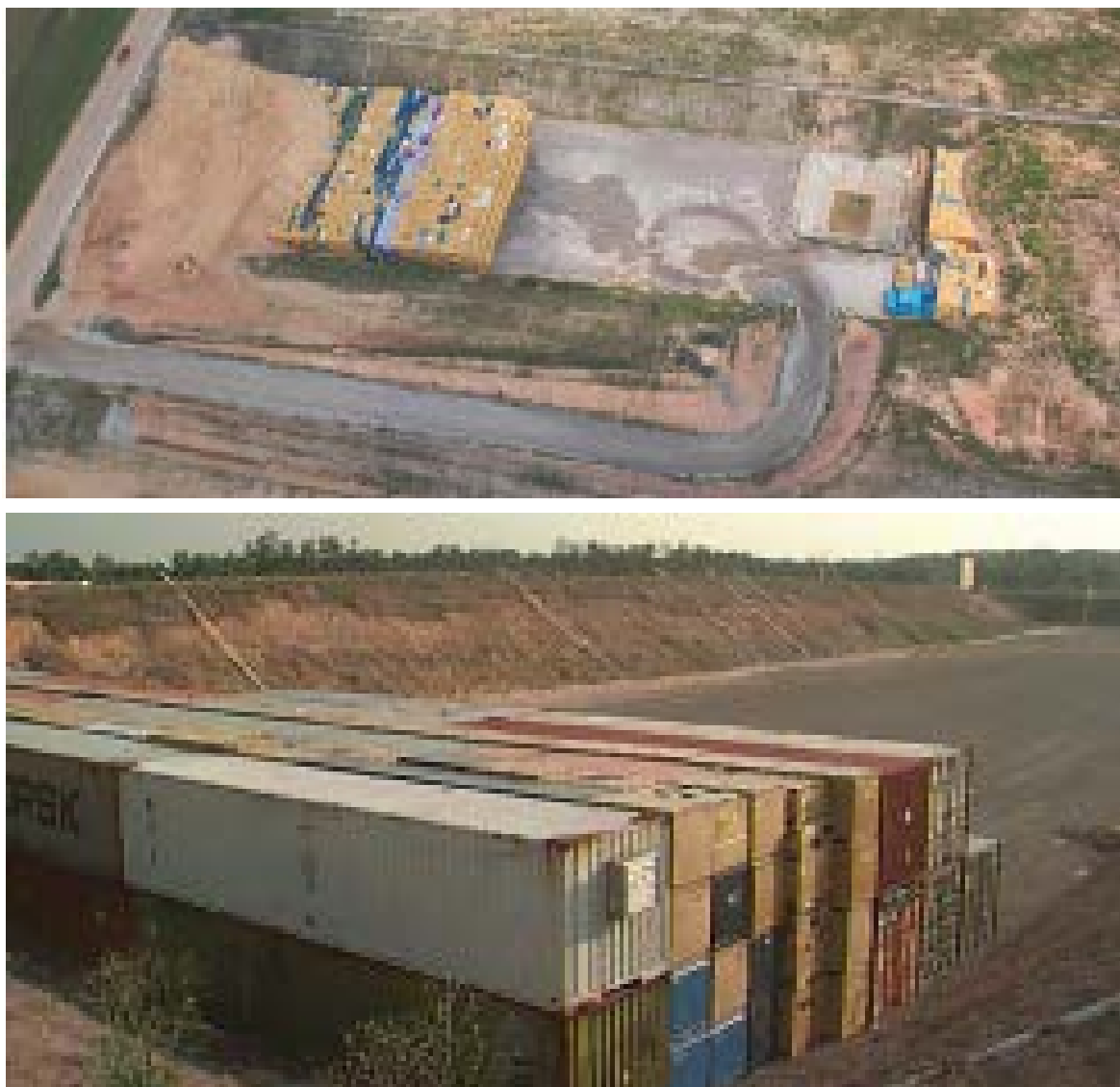
Figure 7. Engineered Trench: (top) aerial view and (bottom) close up of metal containers holding low level waste (WSRC 2008).
