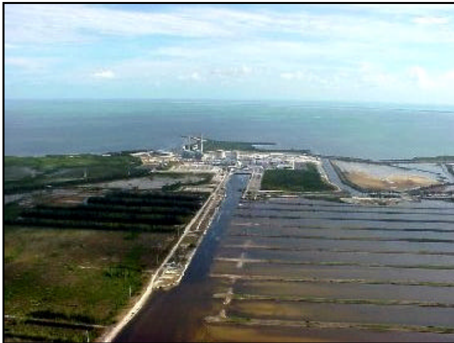
Figure 2. Looking east over cooling canals toward the plant site with Biscayne Bay in the distance.
