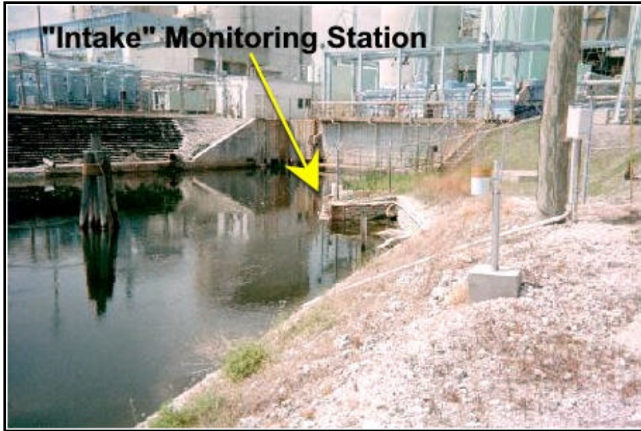
Figure 4. "Intake Site", The water temperature is located within the PVC pipe that extends into the water..
