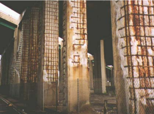
Figure 9: Severely Degraded Bridge Supports
