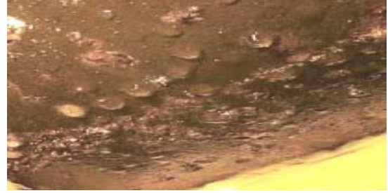
Figure 4: Corrosion Caused by Condensation
