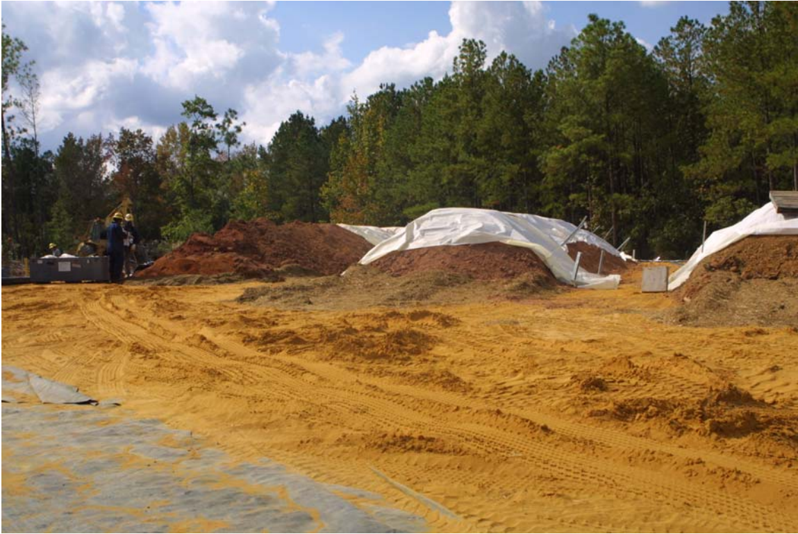
Exhibit 2. Windrows located on the treatment pad near the CMP Pits.
