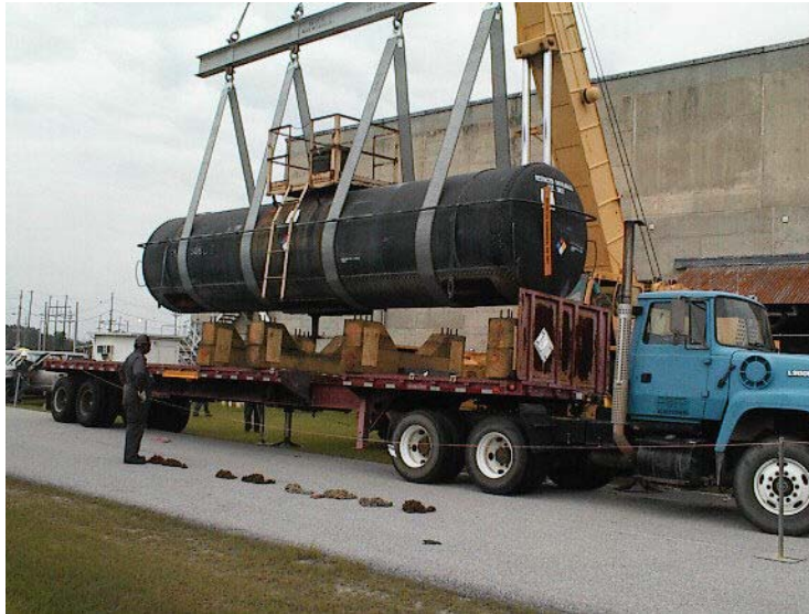
Figure 2. Railcar Tankers lifted from frames onto flatbed trucks
