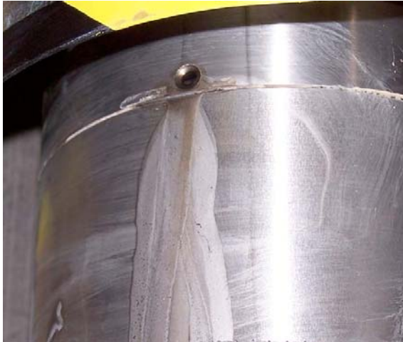
Figure 8 Traces of Filtrate Drips from Rotary Joint Upper Weep Hole
