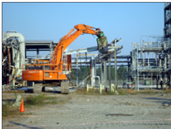
The 100,000-square-foot 247-F complex, located near the rear of F Area, is demolished.
