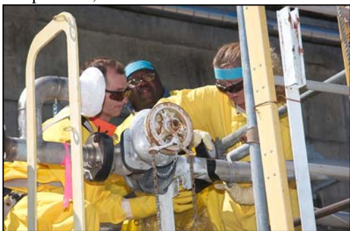
Dawn Manning (right), a member of the Design Lab, installs a glovebag during deactivation work in F Outside Facilities.
