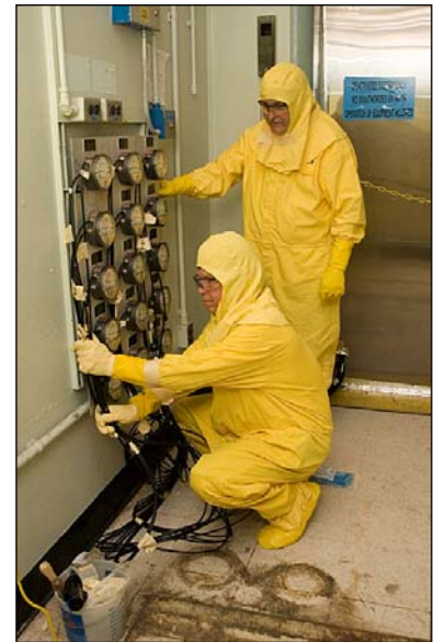
Deactivation workers check final details near the end of FB Line deactivation work.
