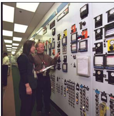
Workers in F Canyon's main control room, which runs the length of the 800-foot-long facility.
