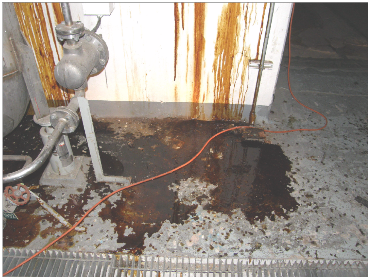
Figure 2 Photograph of sealant that has seeped to the floor next to open grating.
