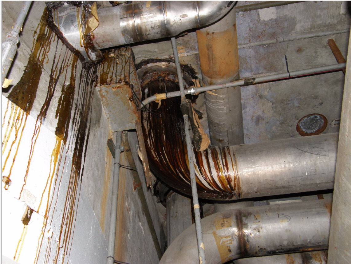
Figure 1. Photograph of degraded sealant leaking from piping penetrations in the reactor biological shield wall.
