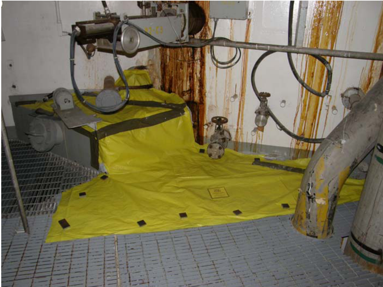
Figure 3. Location in building 105-L at -20 elevation that has been cleaned, covered and labeled. Photo does not show the barricade.
