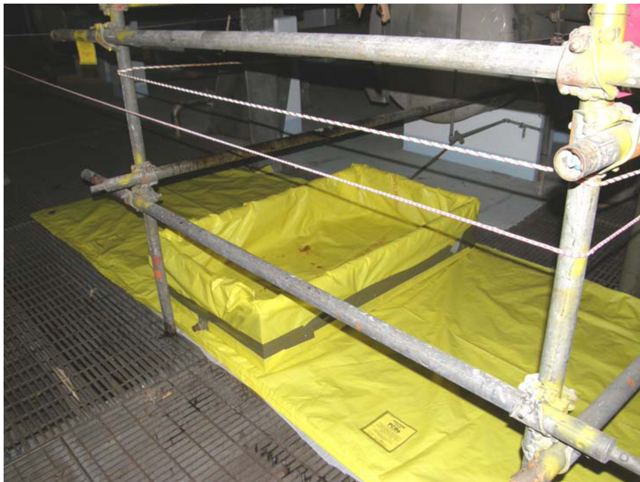
Figure 4. C-Reactor, -20 Elevation location that has been cleaned, covered, labeled and barricaded.
