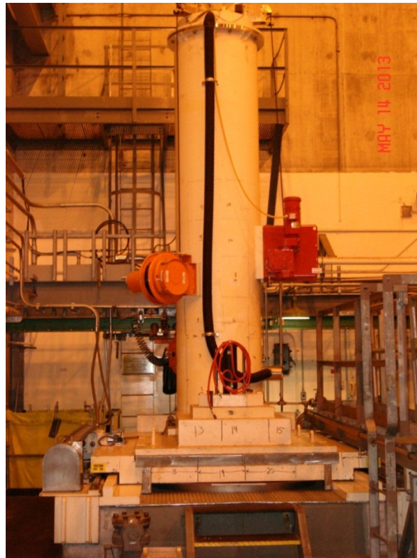
Figure 2-1: Shielded Transfer System (Over Transfer Pit #1)
