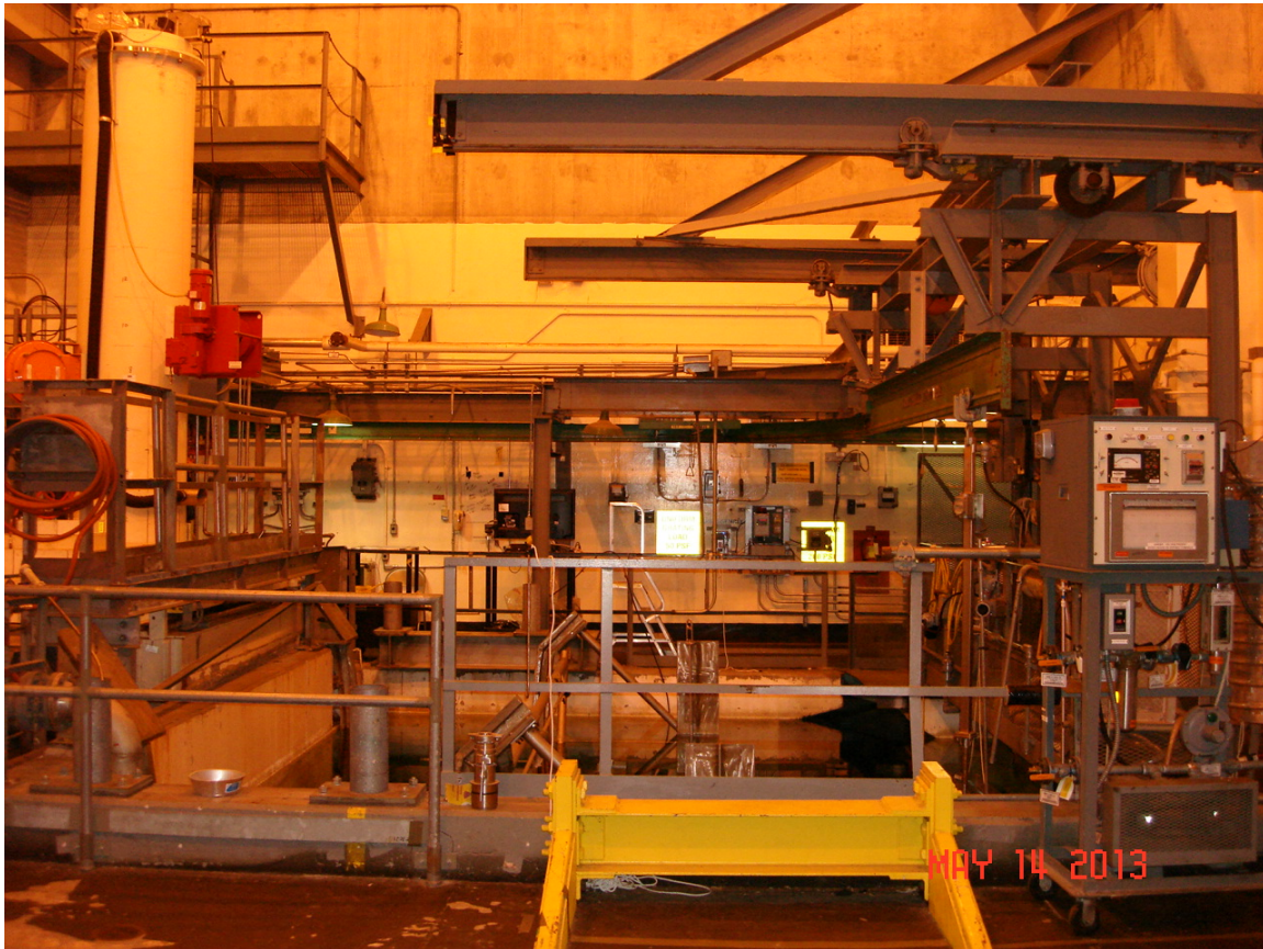
Figure 2-2: View From the East of 105-L Disassembly Area Pit #2 (STS Shield Tube Shown Upper Left)
