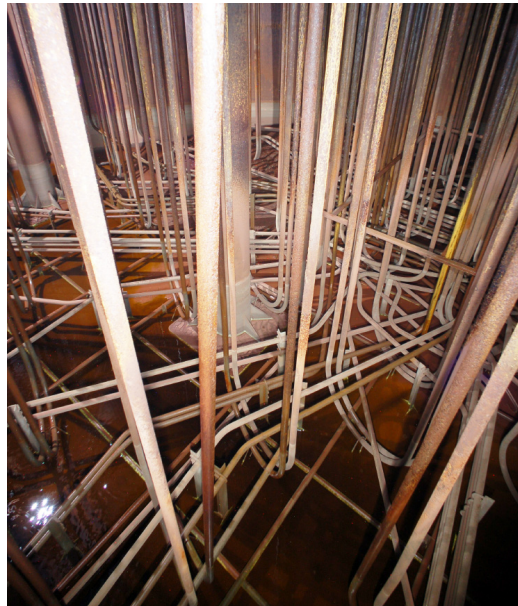
Figure 2. Cooling coils located in the waste tank interior
