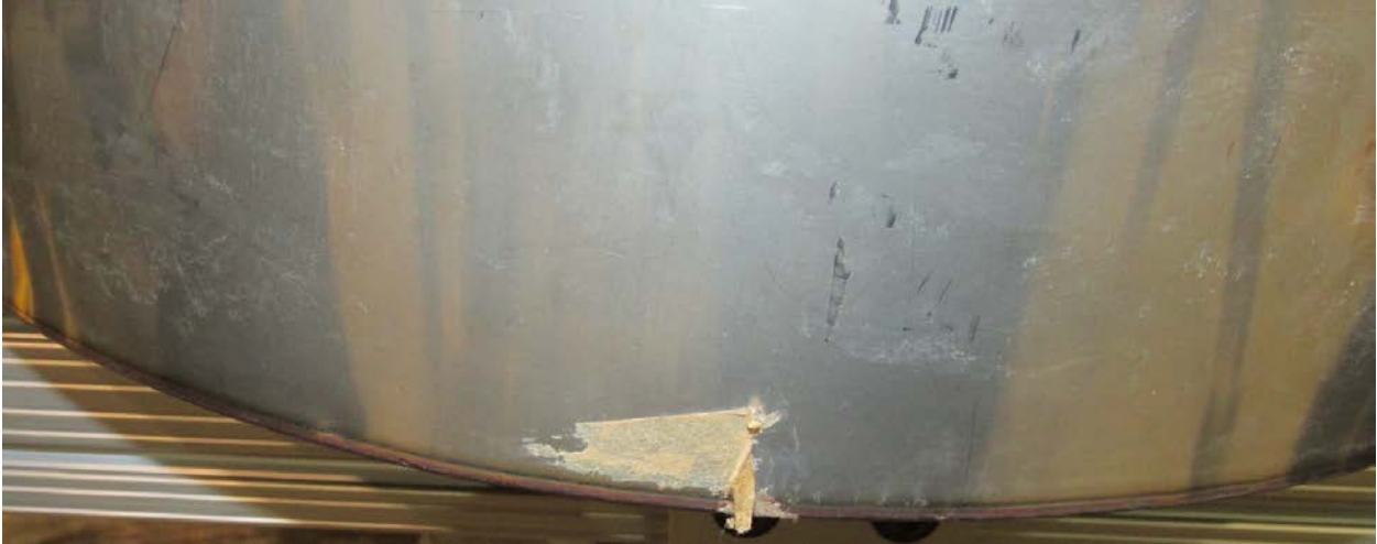
Figure 9. Foreign material on the upper fiberboard assembly air shield, which was identified visually as tape. The upper assembly is upside down in this photo.
