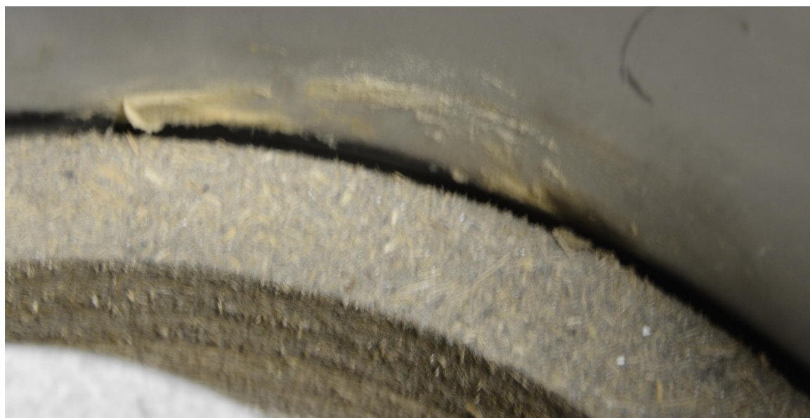
Figure 4. Fibrous deposit on drum interior surface. Photo taken by KAC personnel during surveillance.
