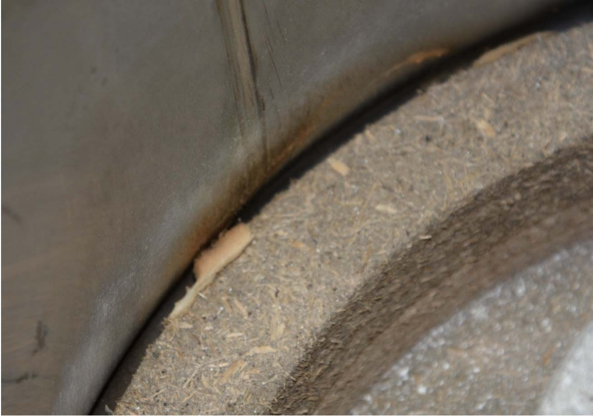
Figure 5. Fibrous deposits on lower fiberboard assembly. Photo taken by KAC personnel during surveillance.
