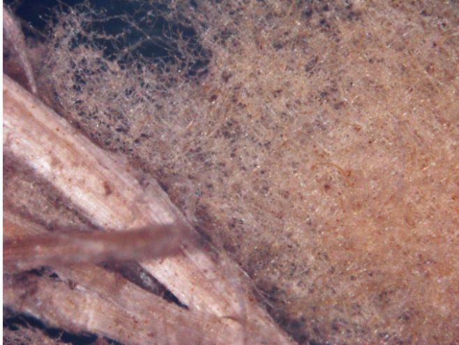
Figure 13. “Fluffy” material removed from the upper fiberboard assembly, photographed at 50X.
