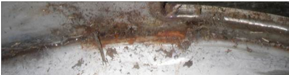
Figure 6. Corrosion of the drum interior along the bottom crevice, observed after 109 weeks in test.
