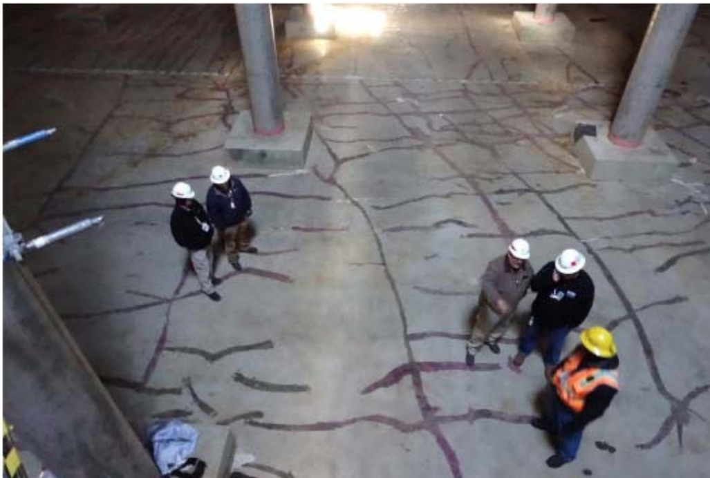
Figure 2. Interior view of SDU6 floor cracking and initial crack sealing attempts [8]
