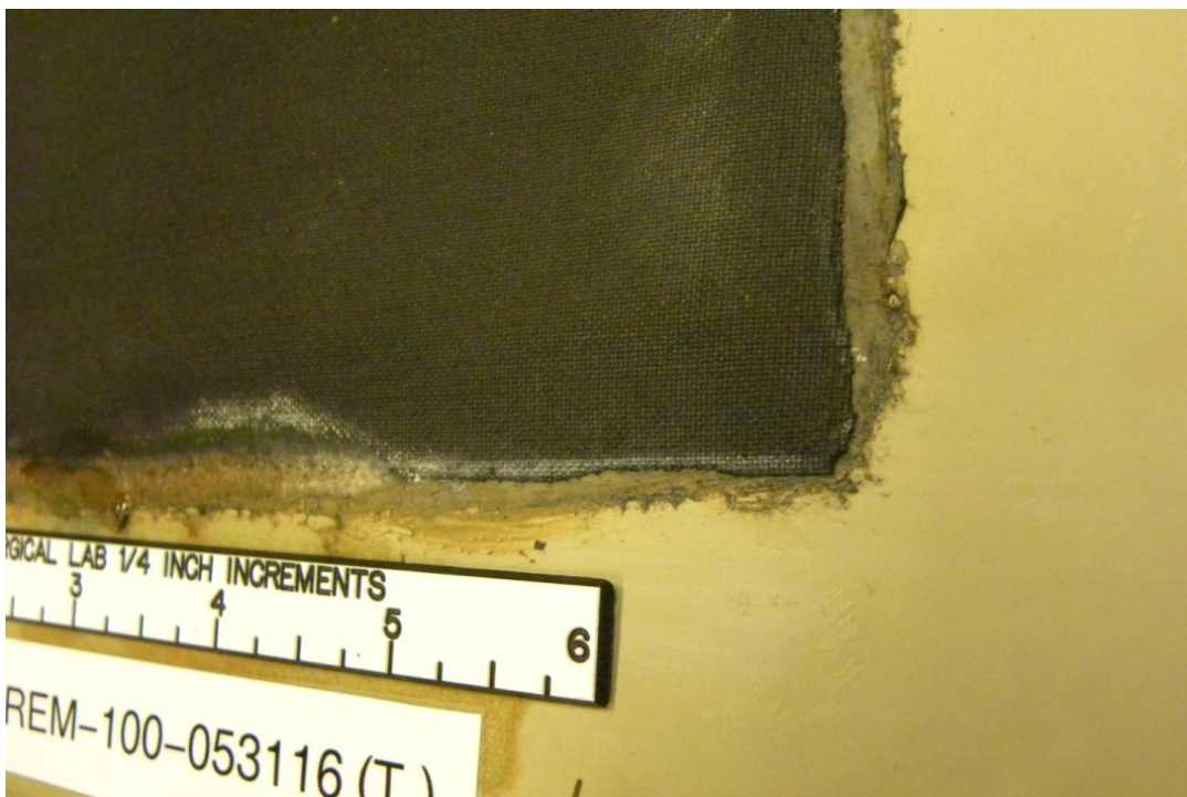
Figure 32. 15SREL-LB-REM-100-053116 (no delamination observed, representative of all corners)
