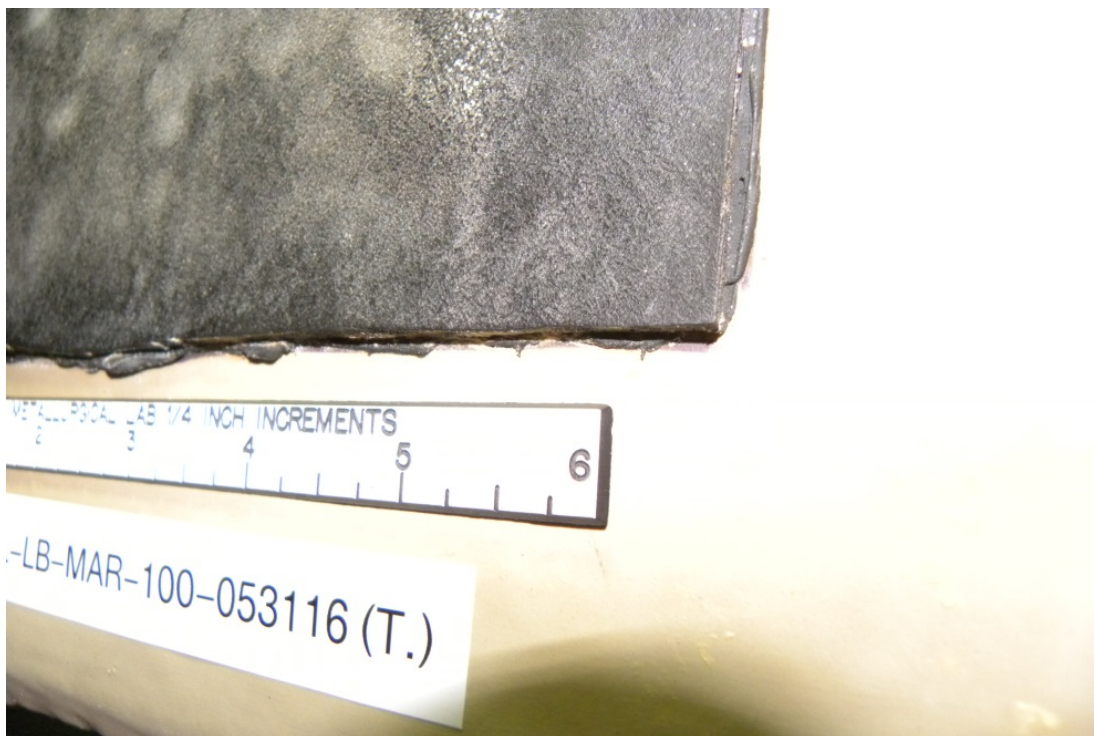
Figure 24. 13SREL-LB-MAR-100-053116 (slight delamination/debonding at corners, as-received, no probing)
