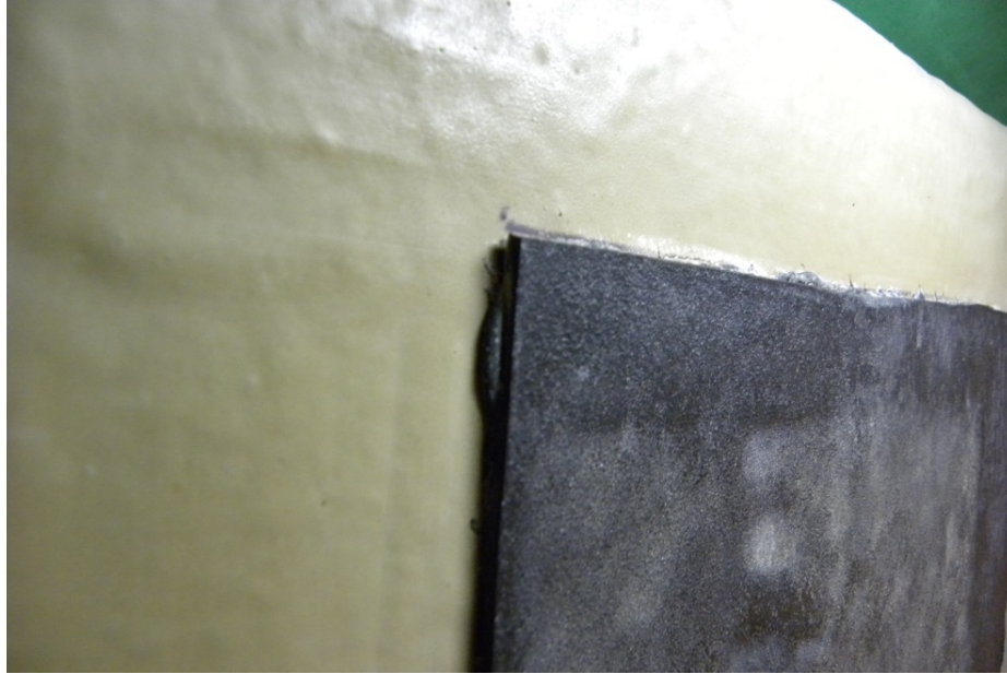
Figure 25. 13SREL-LB-MAR-100-053116 (delamination/debonding at opposite corners, as-received, no probing)
