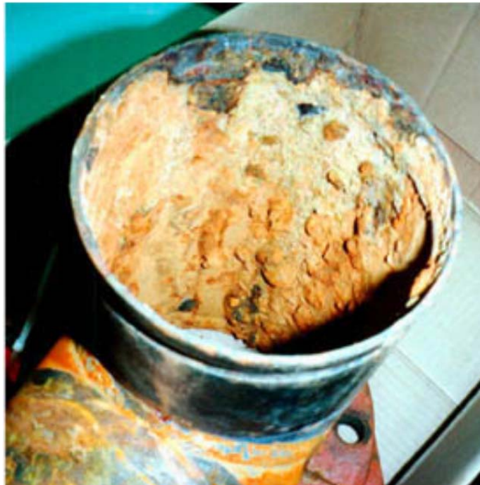
Figure 12. Microbiologically-induced corrosion in a pipe (not SRS piping) [61]
