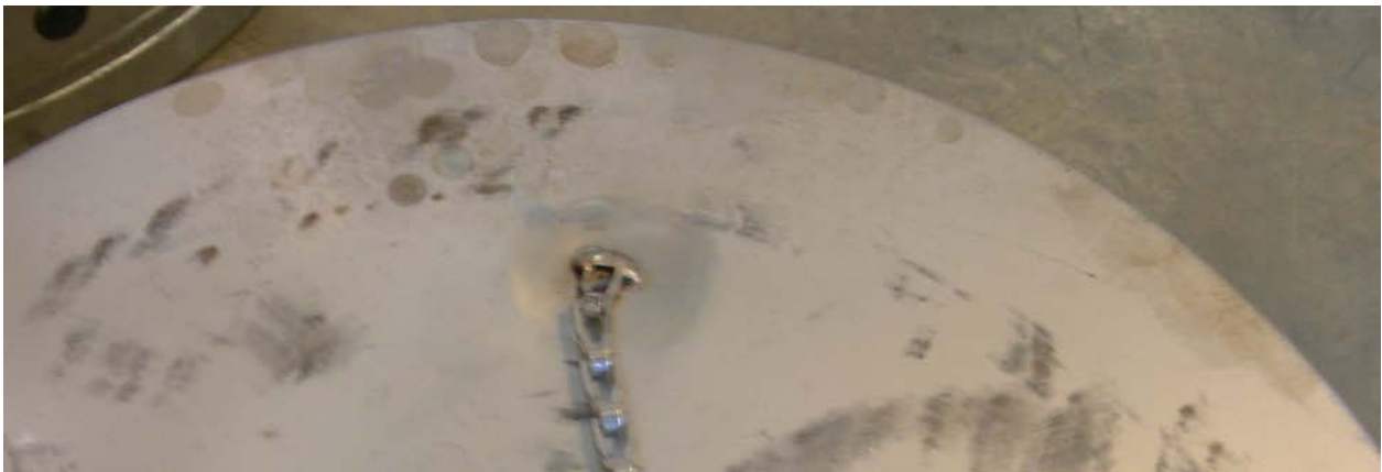
Figure 2. Dried water spots on the 9975-01658 air shield
