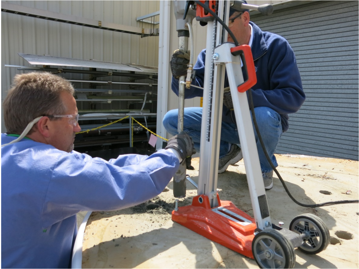
Figure 2-2. Core Drilling Apparatus
