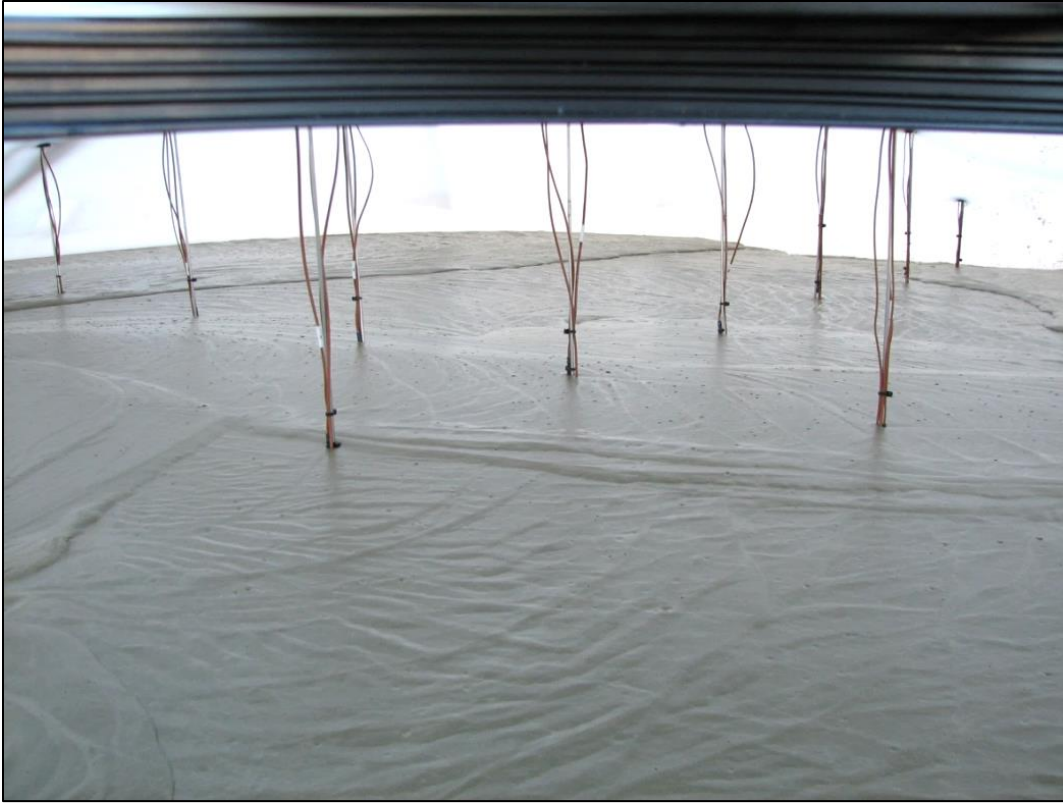
Figure 3-8. Final grout surface after third lift.
