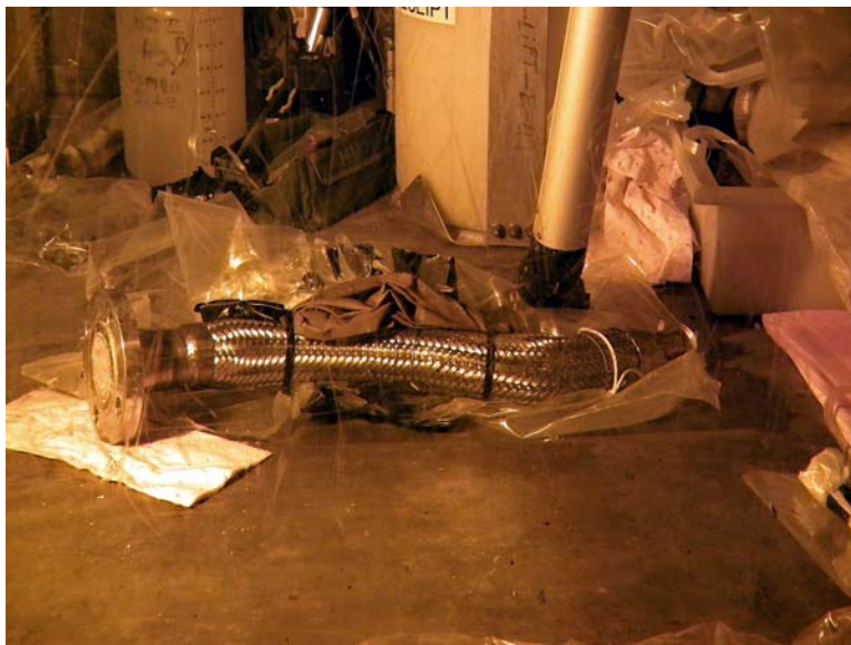
Figure 9. Extraction Contactor #1 Drain line
