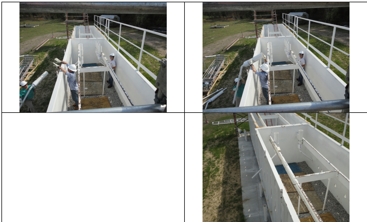
Figure 11 Transfer of secondary housing into roll-off pan (top left and right). The first two secondary housing units in place with effluent plumbing exiting container wall shown (bottom).
