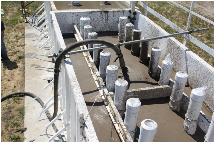
Figure 5 Backfilling the lysimeter pans with CLSM
