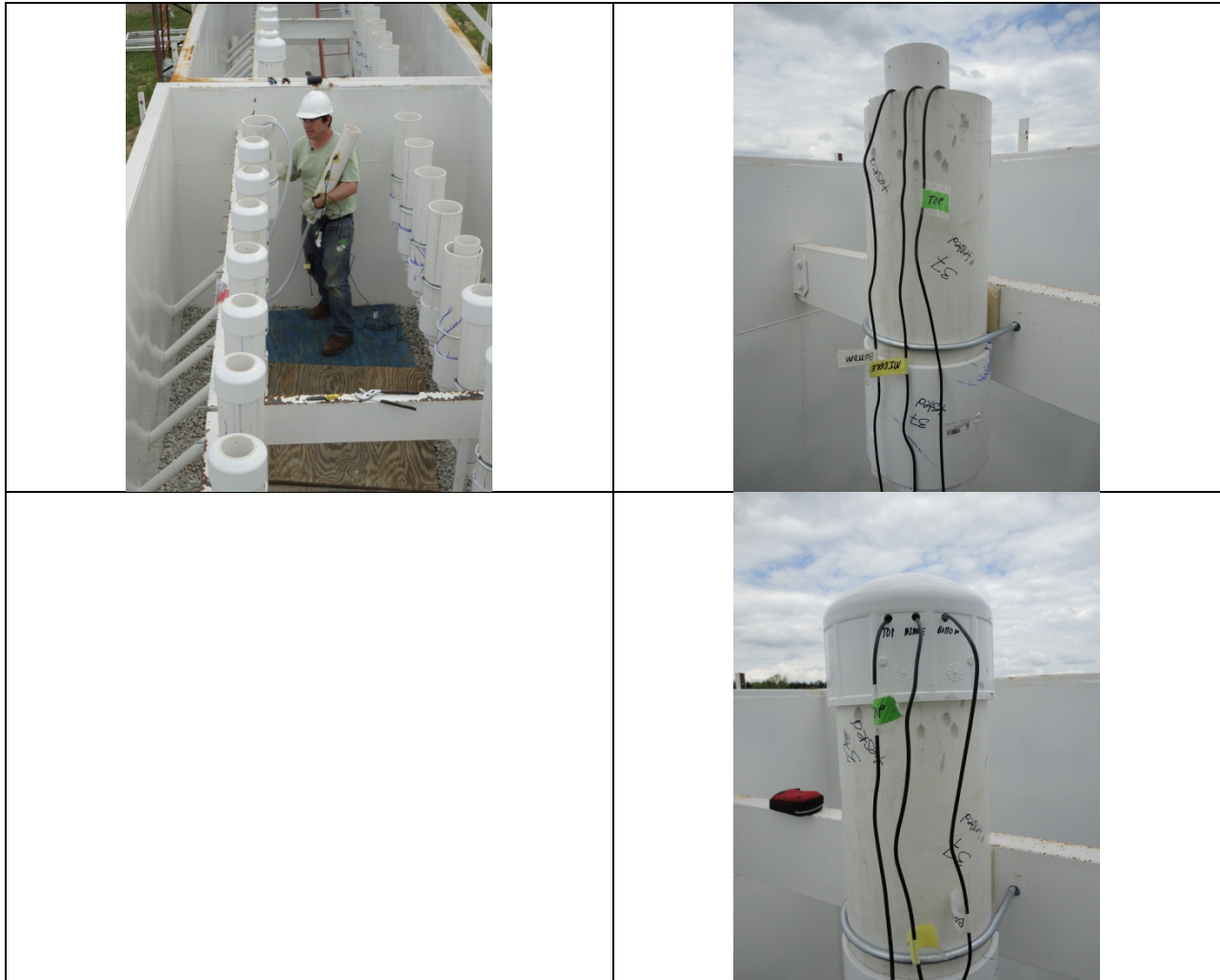
Figure 13 Installation of control lysimeters. Top right photo shows wires coming out the top of the 8" diameter secondary housing. The bottom right photo shows the cap installed with the wires coming out of the respective holes. The wires were stored in the secondary housing for protection.
