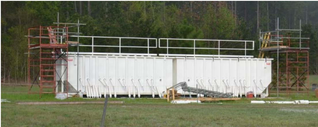
Figure 4 Lysimeter facility during construction with scaffolding for access to container interior
