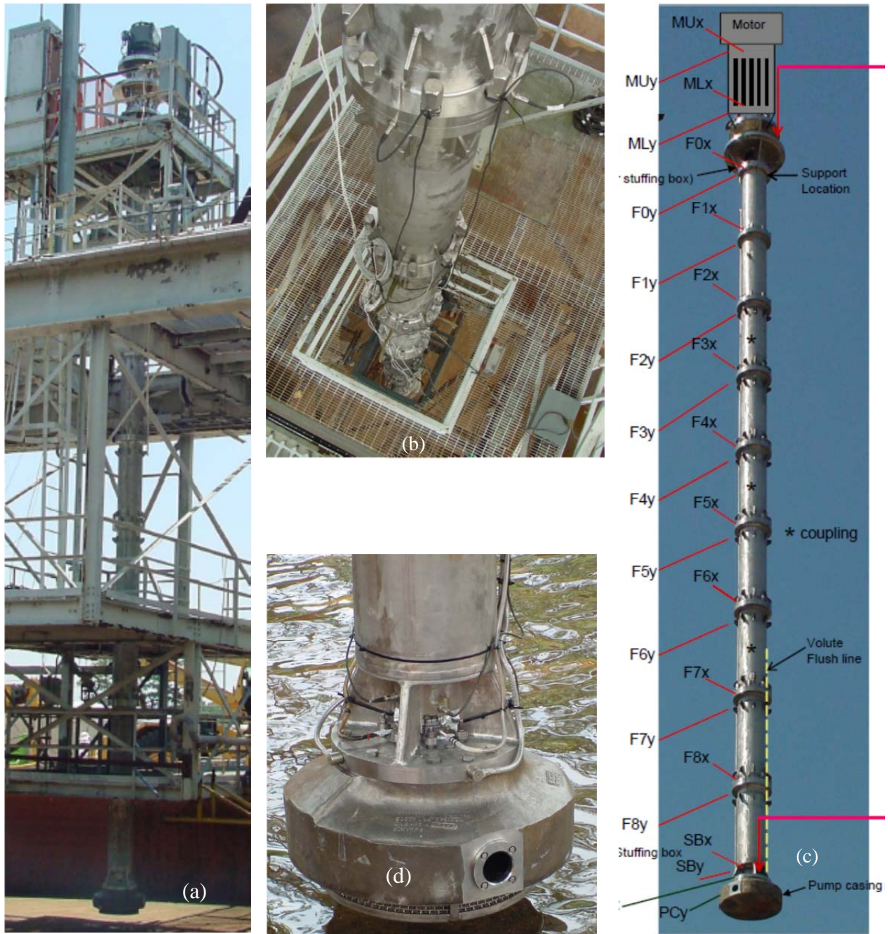
Figure 4. Typical SRS long-shaft pump instrumented with vibration sensors during pre-deployment testing.
