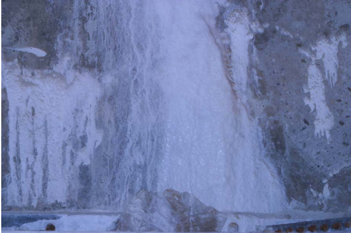
Figure 18 Build-up Deposits of Calcium Carbonate due to Leakage Through Minor Cracks in L Basin [photograph April 2010]
