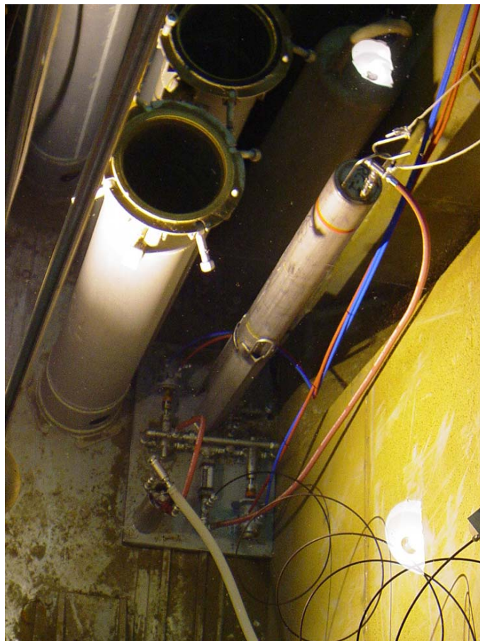
Figure 12. RBOF Underwater deionizer with Empty Oversized Canister Bottom Halves
