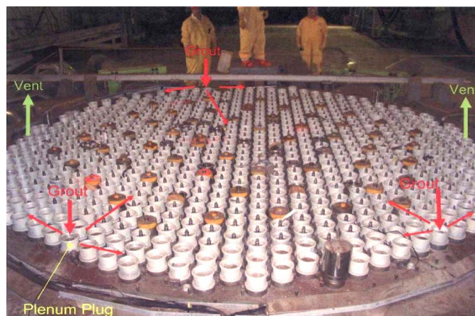
Figure 9. Top of the P-Reactor plenum.
