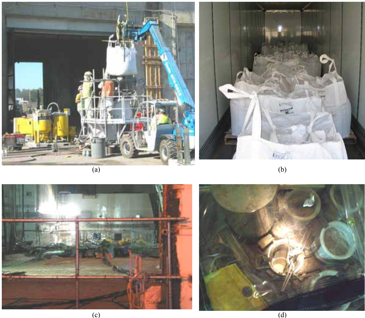
Figure 11. P-Reactor Vessel ISD.
