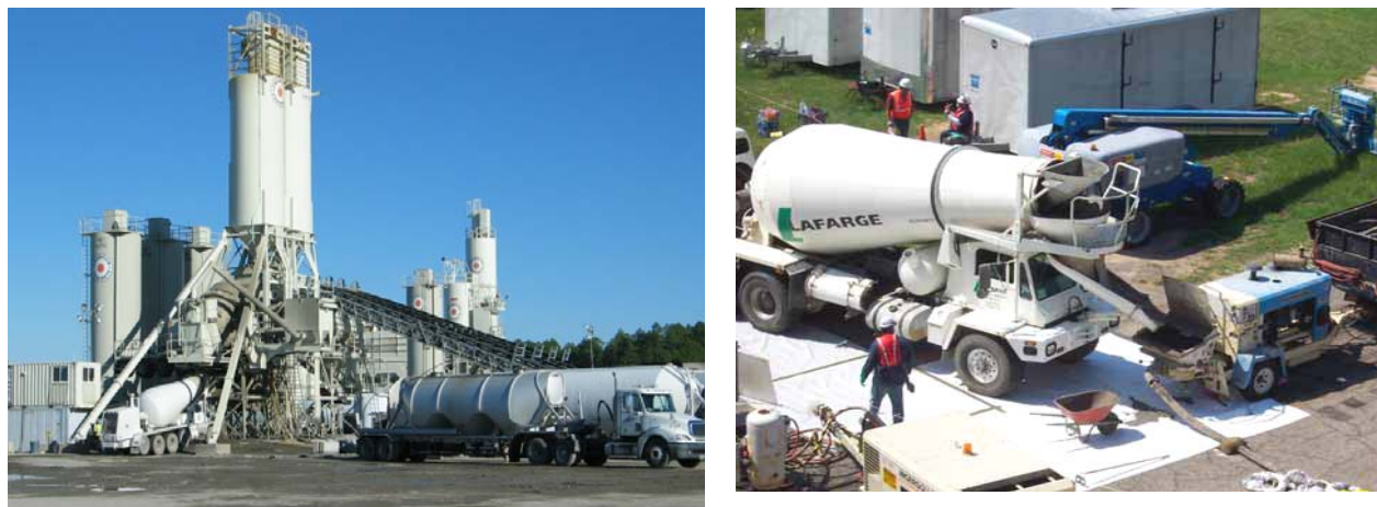
Figure 4. Two On-site concrete batch plants located in P-Area used to produce ISD fill (left) and delivery and pumping of ISD grout in the R-Reactor Disassembly Basin (right).
