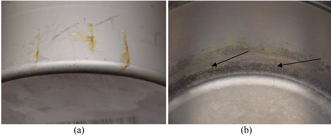
Figure 3. Bottom of as-fabricated 3013 outer container after boiling Magnesium Chloride test: a) Exterior through wall cracks; b) Interior cracks, arrows indicate cracks
