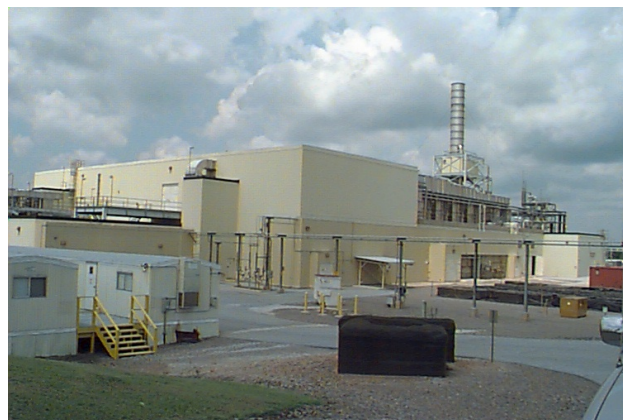
Fig. 2. Building 247-F prior to deactivation, seen from the southwest.
