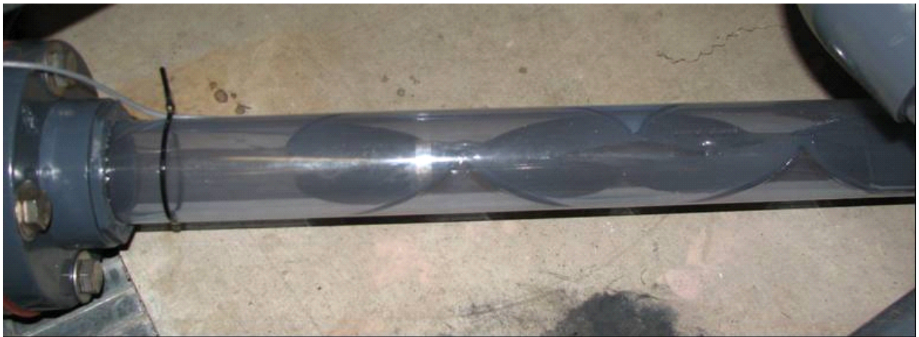
Figure 5: Installed Static Mixer
