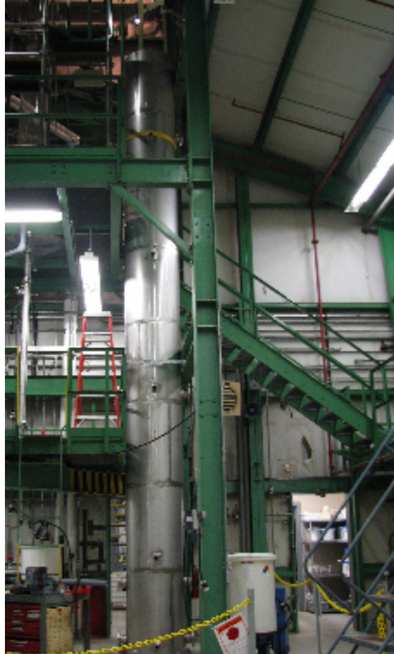
Figure 1: Column Installation for Water and AZ101 Testing
