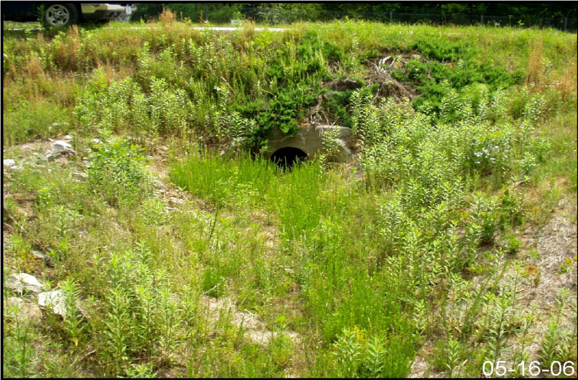
Figure 2-129. View of Storm Water Outfall Z-03.
