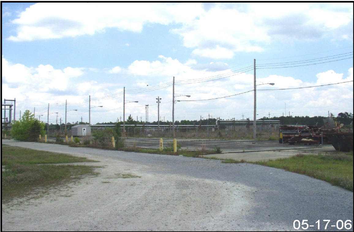
Figure 2-112. Representative View of Drainage Area for Storm Water Outfall P-07.
