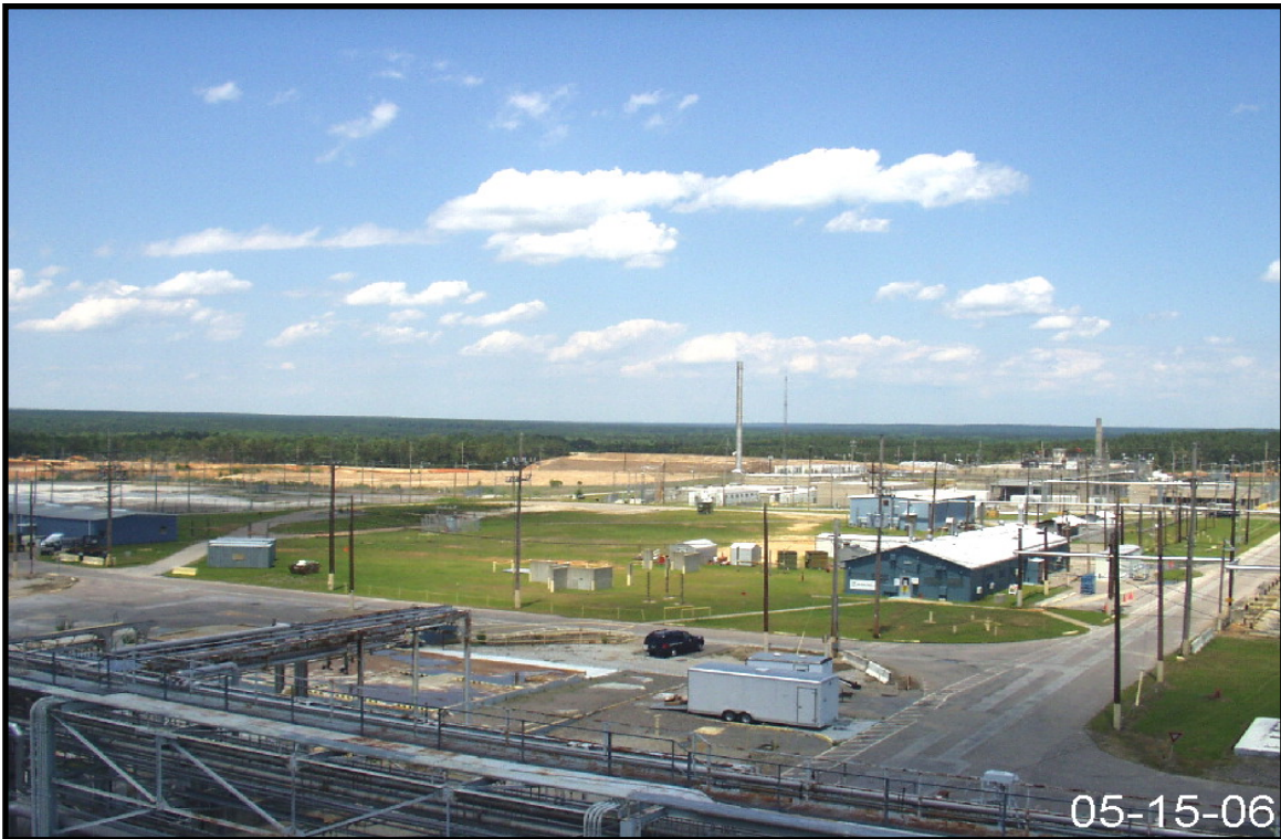
Figure 2-34. Representative View of Drainage Area for Storm Water Outfall F-3B.
