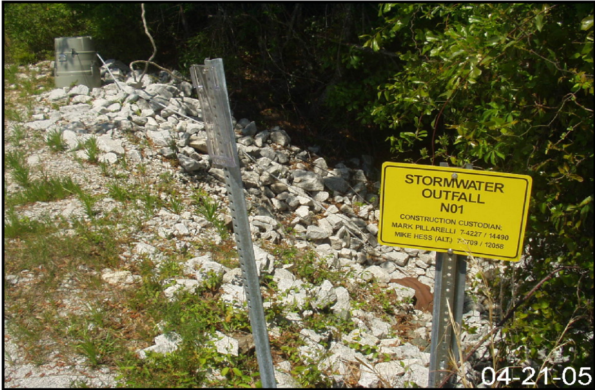
Figure 2-71. View of Storm Water Outfall N-01.
