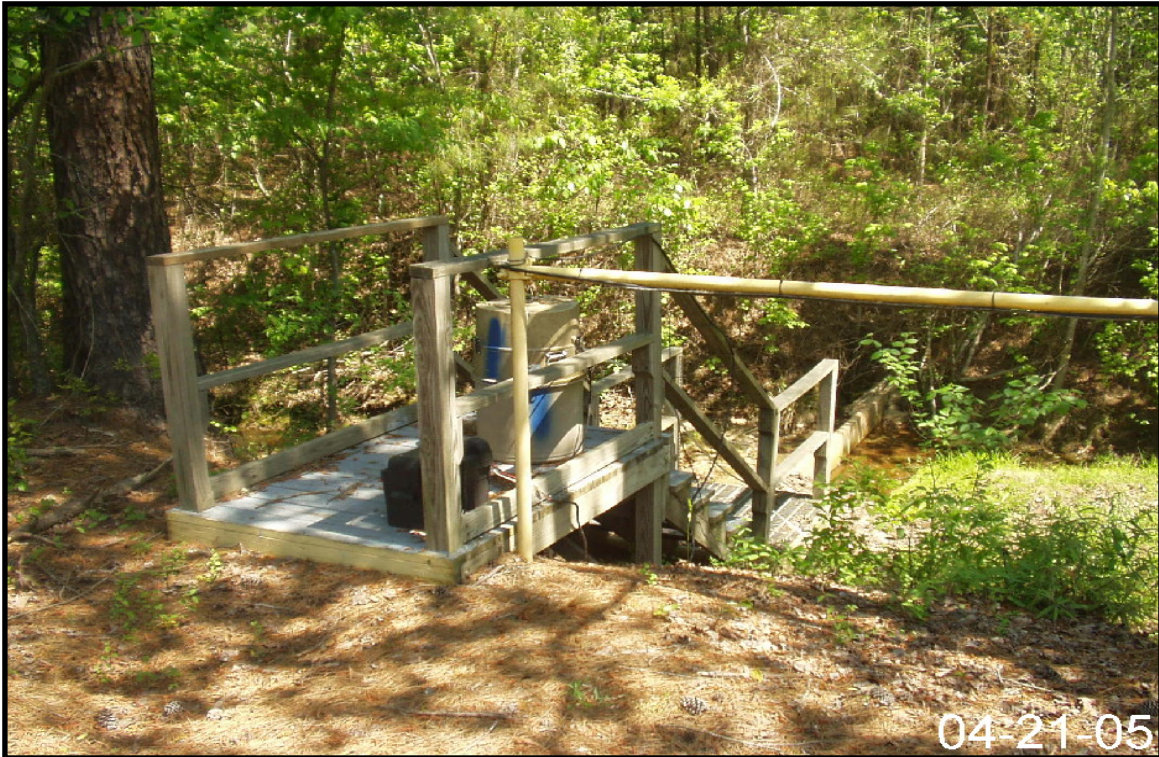
Figure 2-87. View of Storm Water Outfall N-06.
