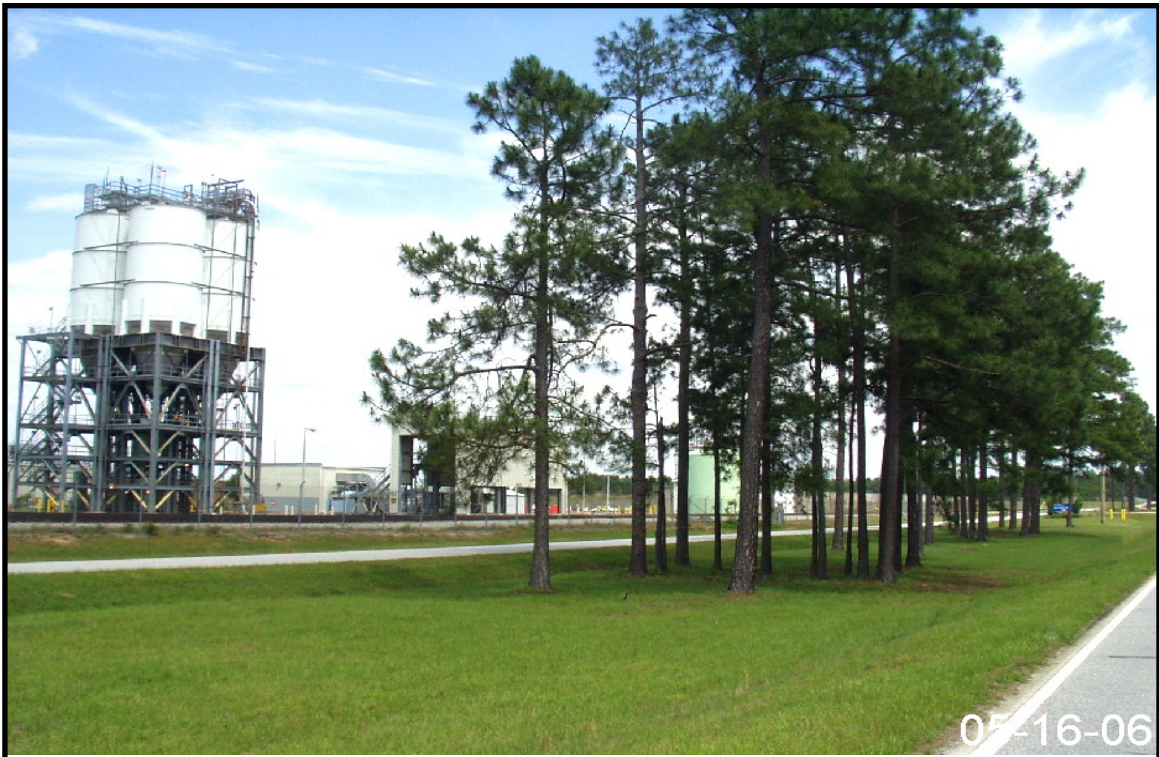
Figure 2-127. Representative View of Drainage Area for Storm Water Outfall Z-01.
