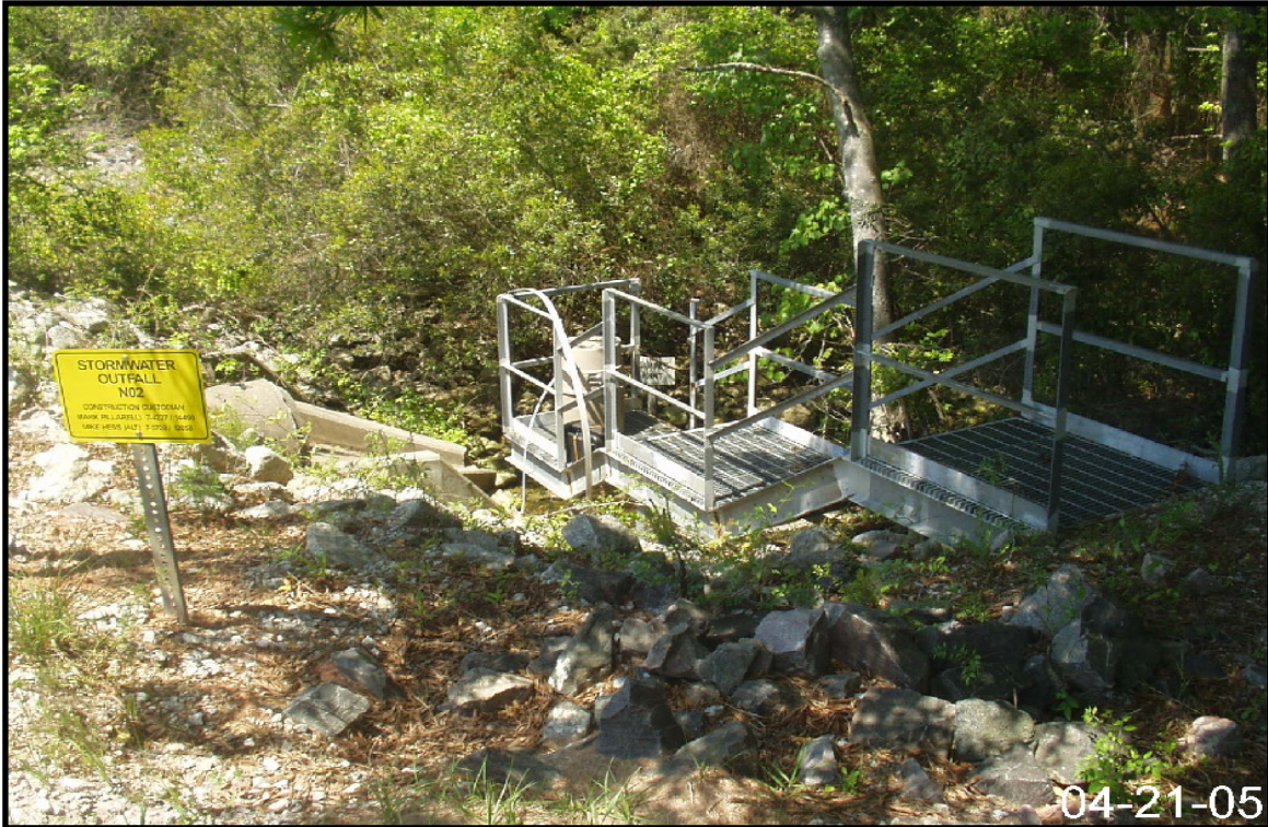
Figure 2-75. View of Storm Water Outfall N-02.
