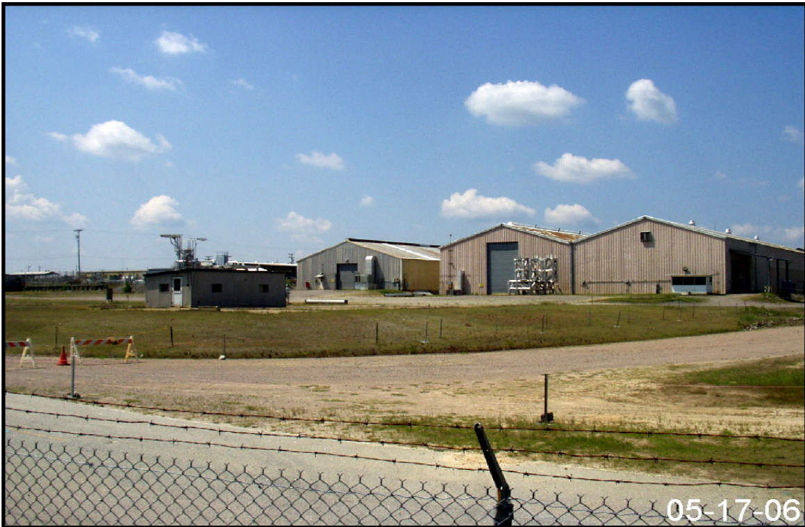
Figure 2-79. Representative View of Drainage Area for Storm Water Outfall N-2A.
