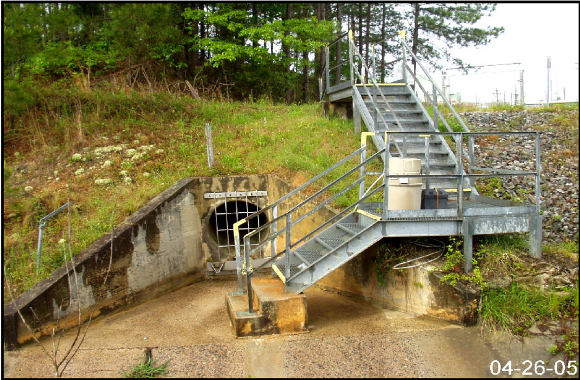
Figure 2-39. View of Storm Water Outfall H-06.
