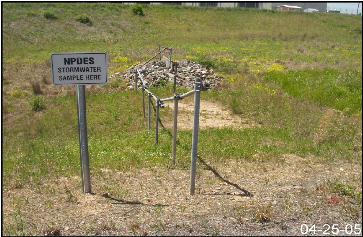
Figure 2-21. View of Storm Water Outfall E-03.
