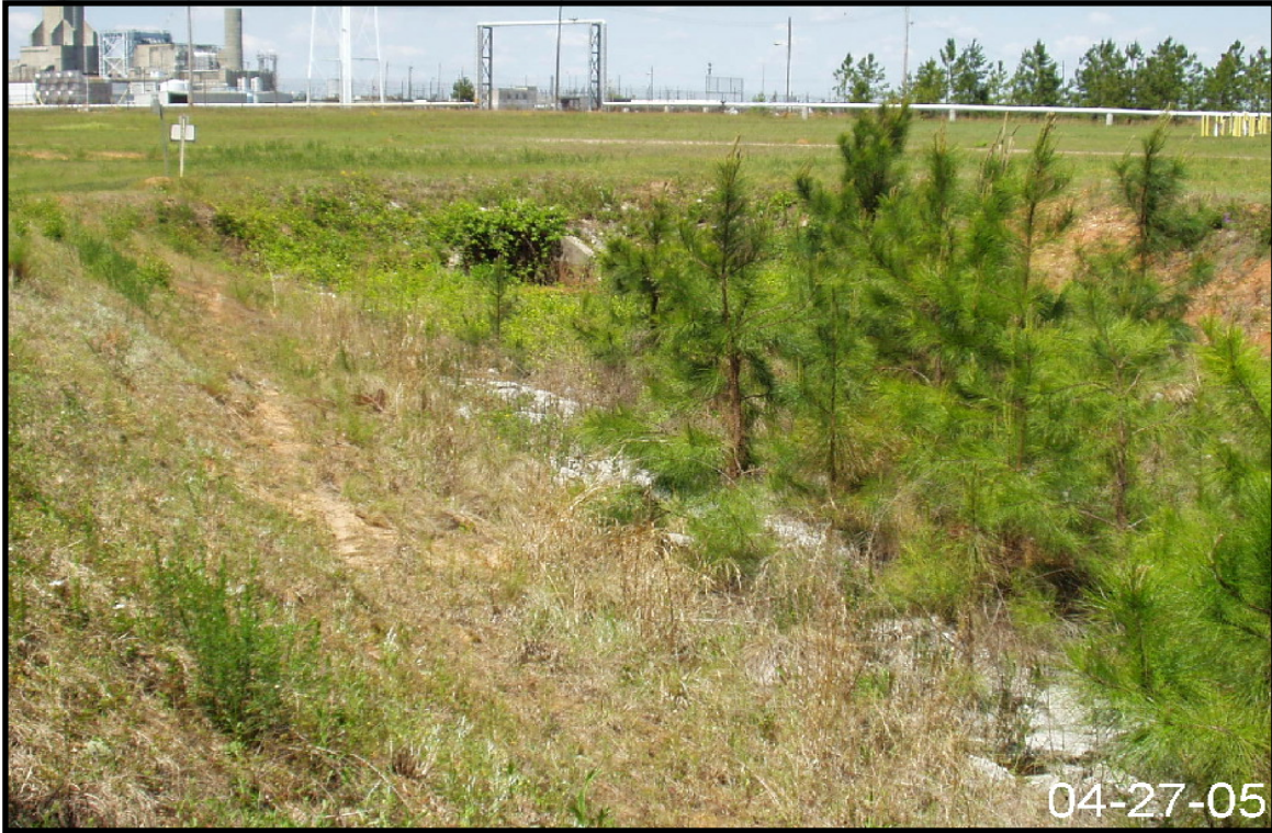
Figure 2-59. View of Storm Water Outfall K-04.
