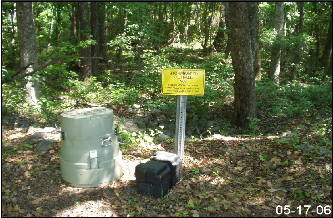
Figure 2-81. View of Storm Water Outfall N-03.
