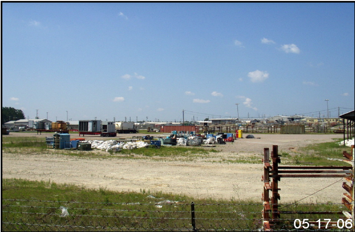
Figure 2-85. Representative View of Drainage Area for Storm Water Outfall N-05.
