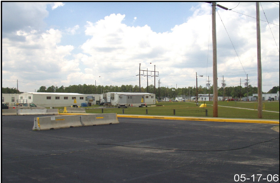
Figure 2-66. Representative View of Drainage Area for Storm Water Outfall L-09.
