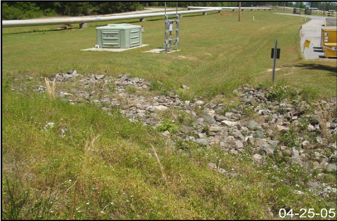
Figure 2-36. View of Storm Water Outfall FT-01.
