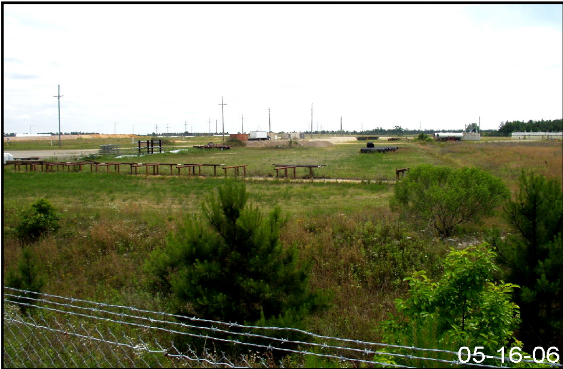
Figure 2-25. Representative View of Drainage Area for Storm Water Outfall E-04.
