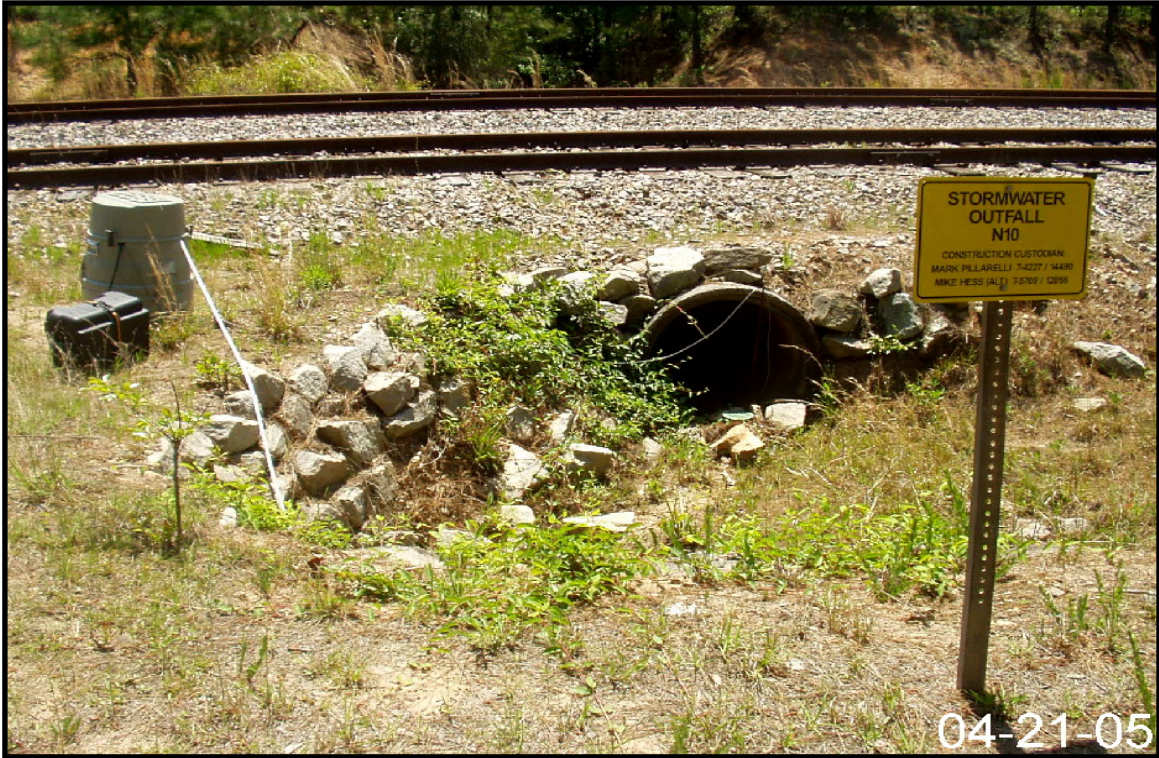
Figure 2-90. View of Storm Water Outfall N-10.
