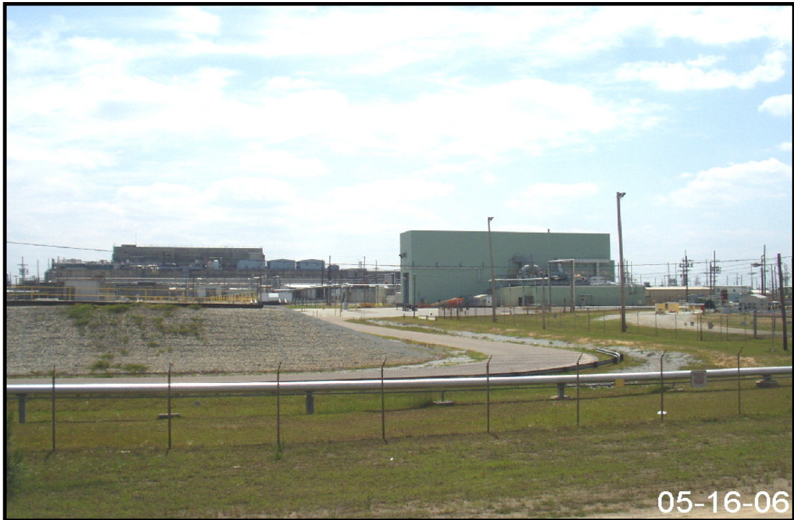
Figure 2-40. Representative View of Drainage Area for Storm Water Outfall H-06.
