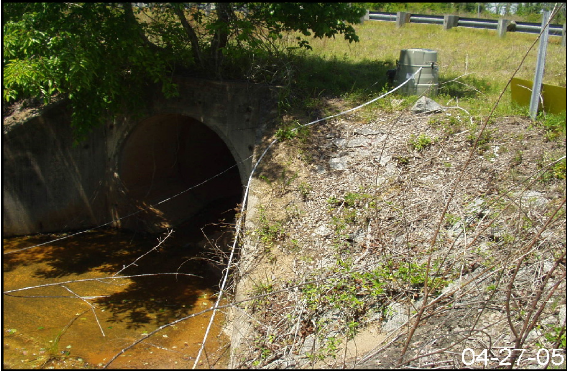
Figure 2-62. View of Storm Water Outfall L-03.
