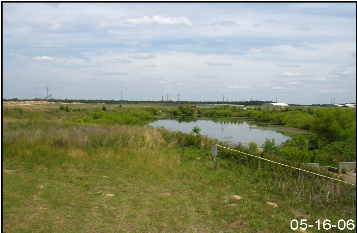
Figure 2-19. Representative View of Drainage Area for Storm Water Outfall E-02.
