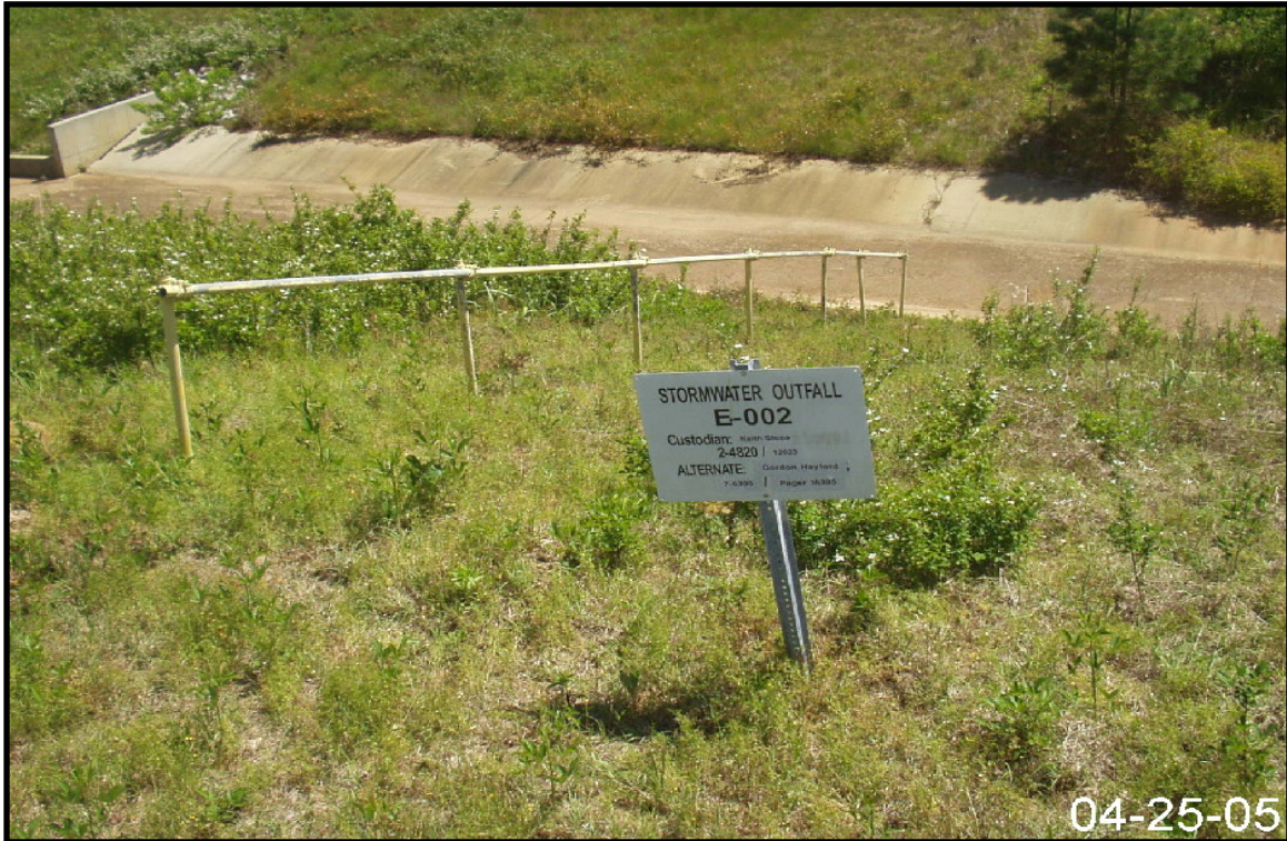
Figure 2-18. View of Storm Water Outfall E-02.
