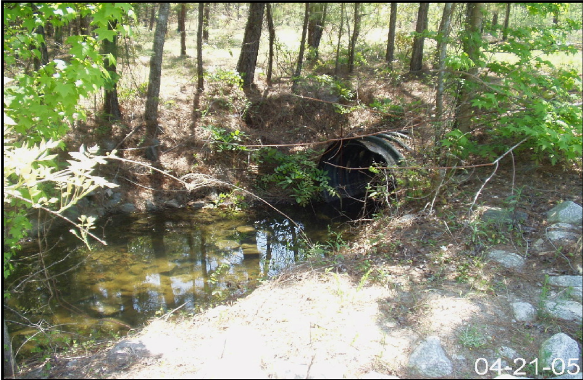
Figure 2-108. View of Storm Water Outfall N-16.
