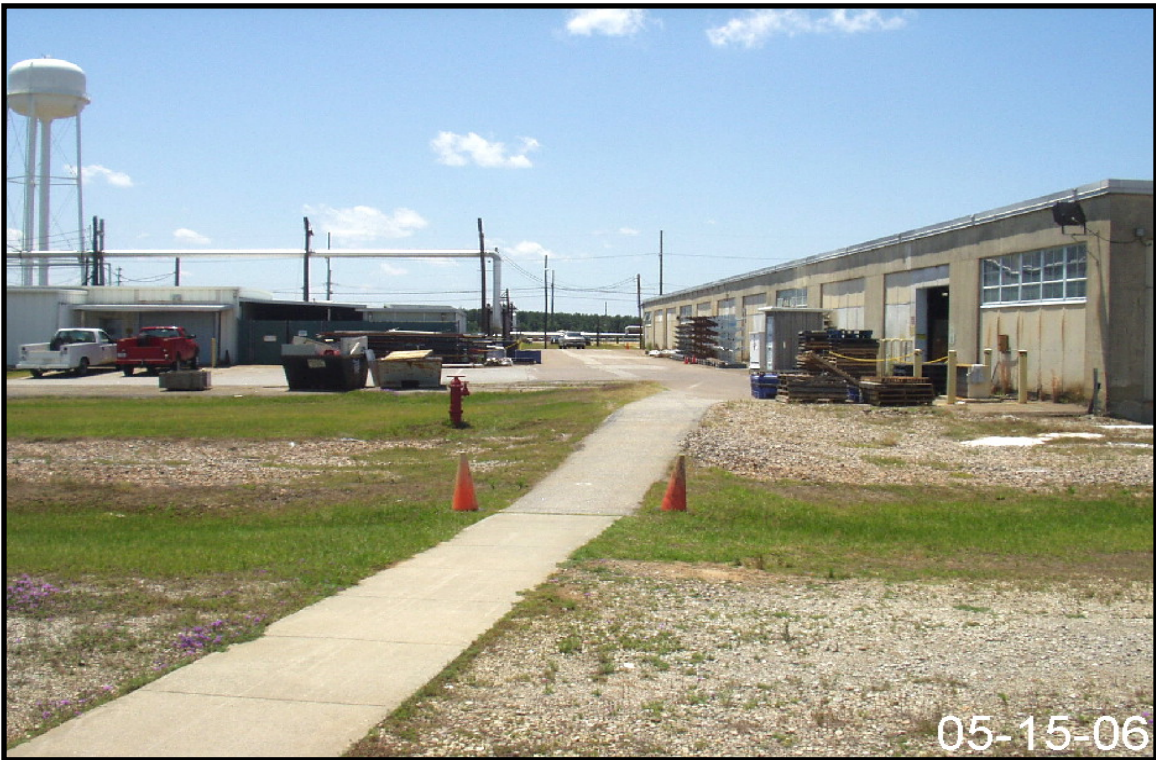
Figure 2-4. Representative View of Drainage Area for Storm Water Outfall A-08.
