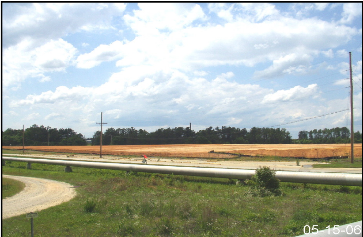
Figure 2-28. Representative View of Drainage Area for Storm Water Outfall E-05.
