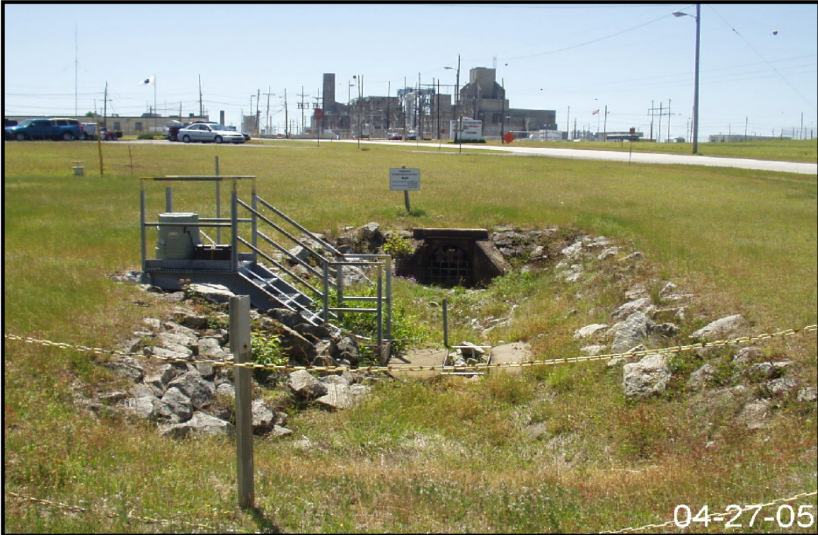
Figure 2-51. View of Storm Water Outfall K-01.
