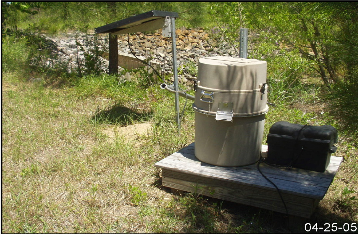
Figure 2-27. View of Storm Water Outfall E-05.
