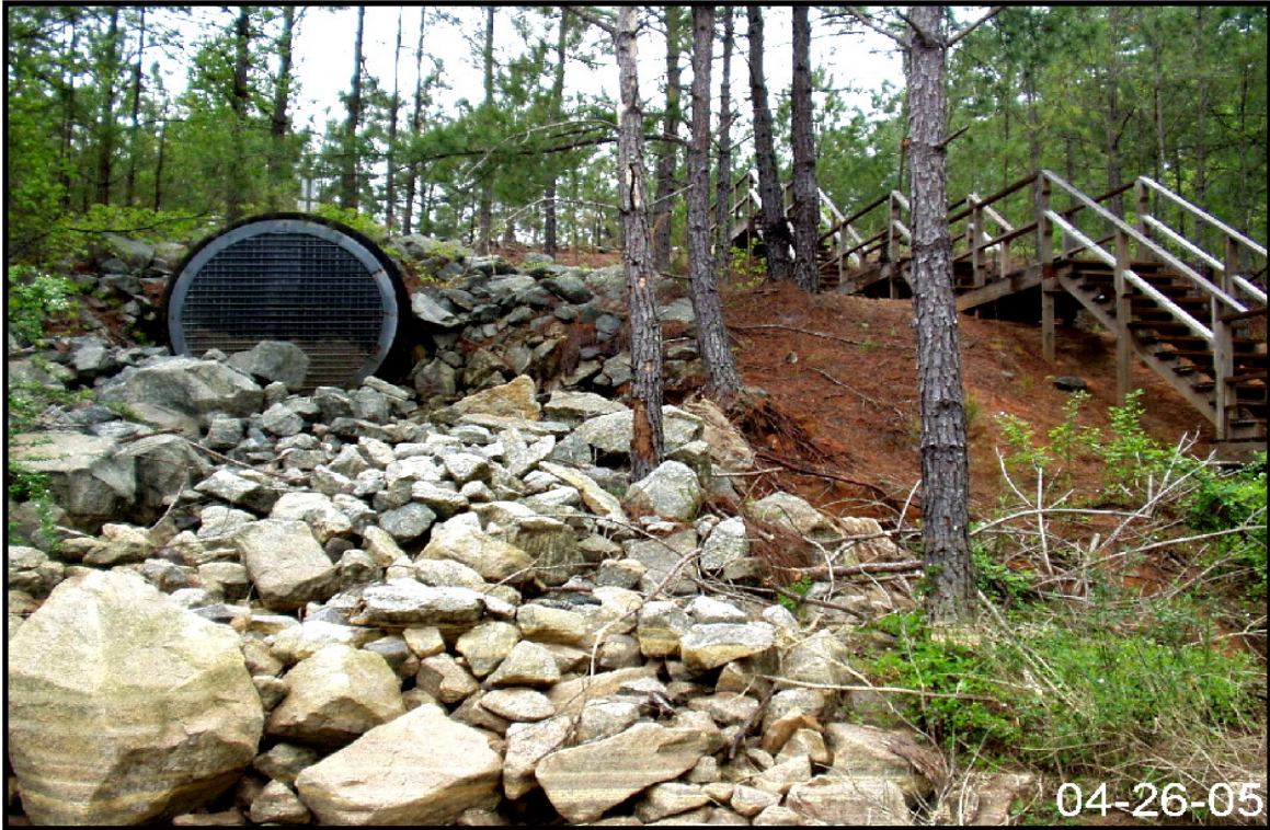
Figure 2-126. View of Storm Water Outfall Z-01.
