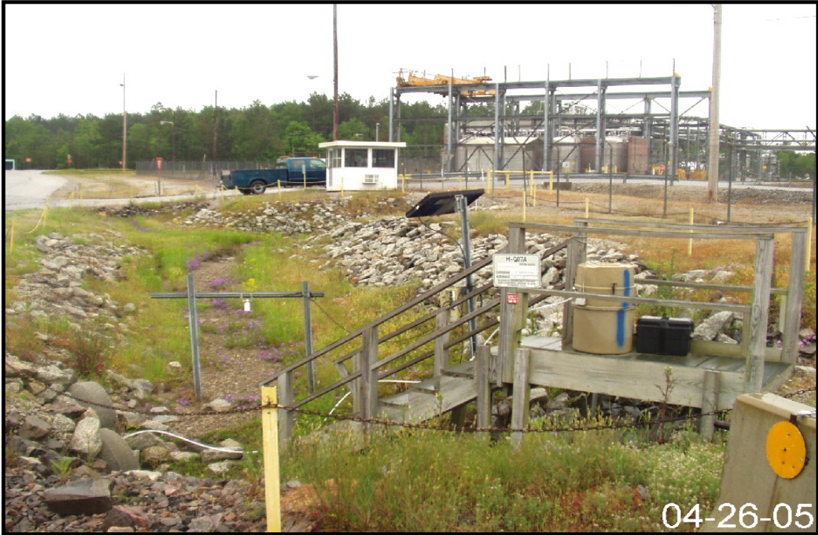
Figure 2-42. View of Storm Water Outfall H-7A.
