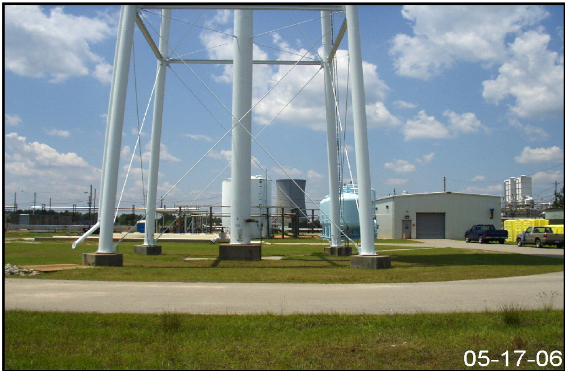
Figure 2-60. Partial View of Drainage Area for Storm Water Outfall K-04.
