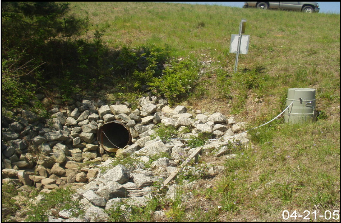
Figure 2-33. View of Storm Water Outfall F-3B.
