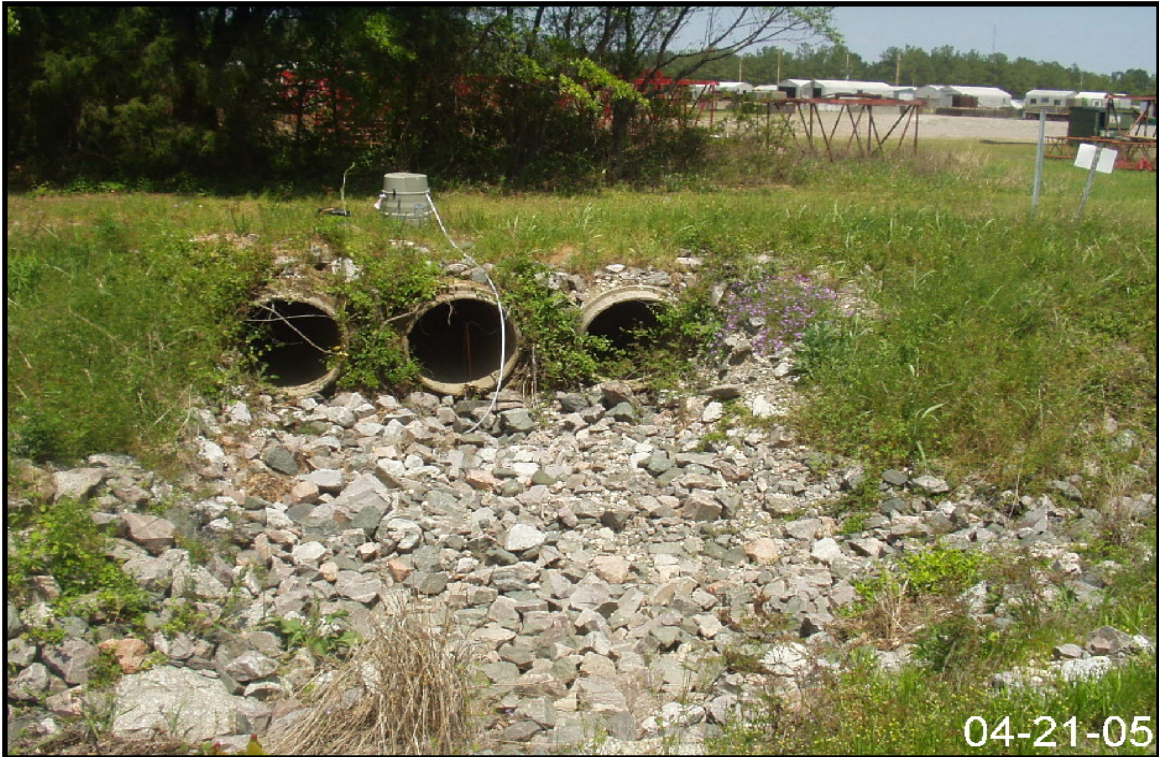
Figure 2-93. View of Storm Water Outfall N-12.
