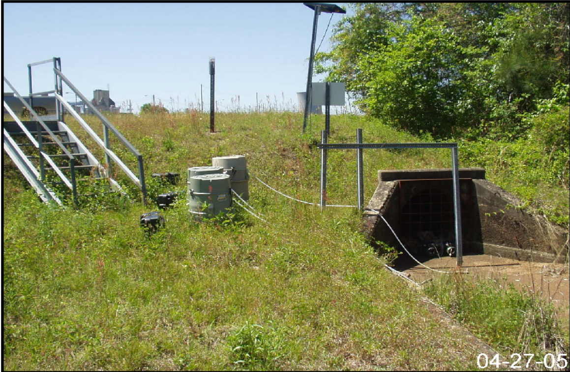
Figure 2-55. View of Storm Water Outfall K-02.
