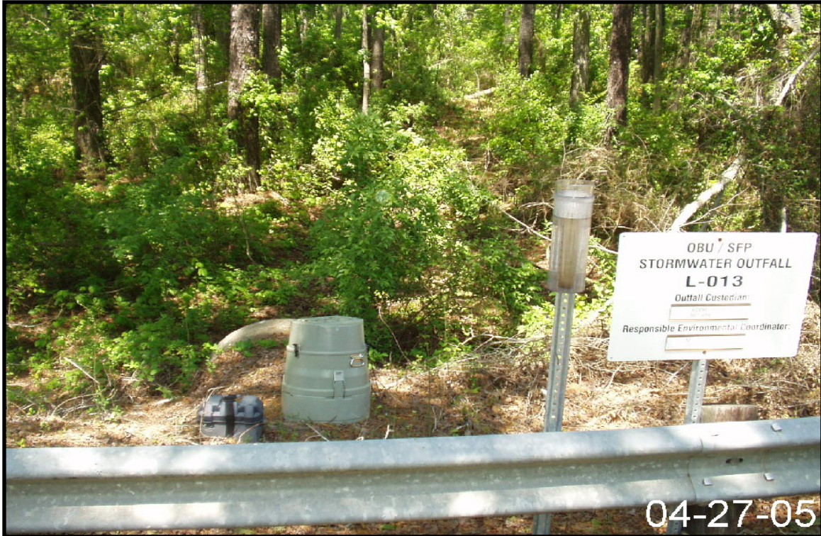
Figure 2-68. View of Storm Water Outfall L-13.
