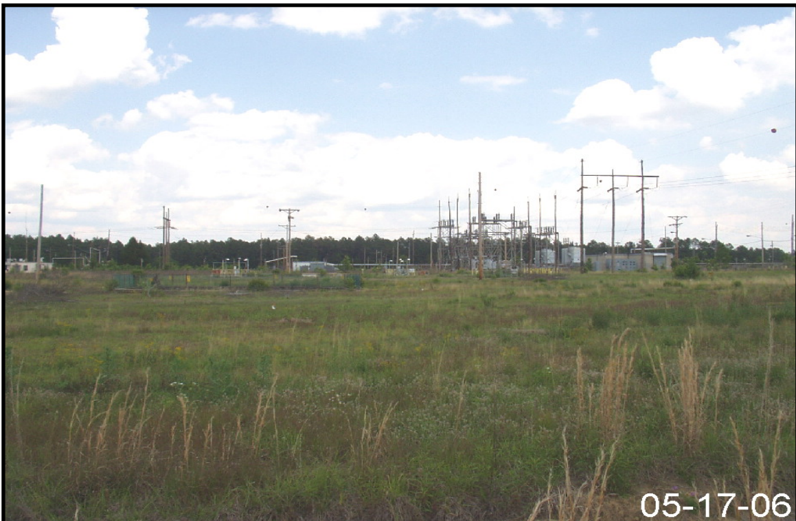
Figure 2-115. Representative View of Drainage Area for Storm water Outfall P-13.
