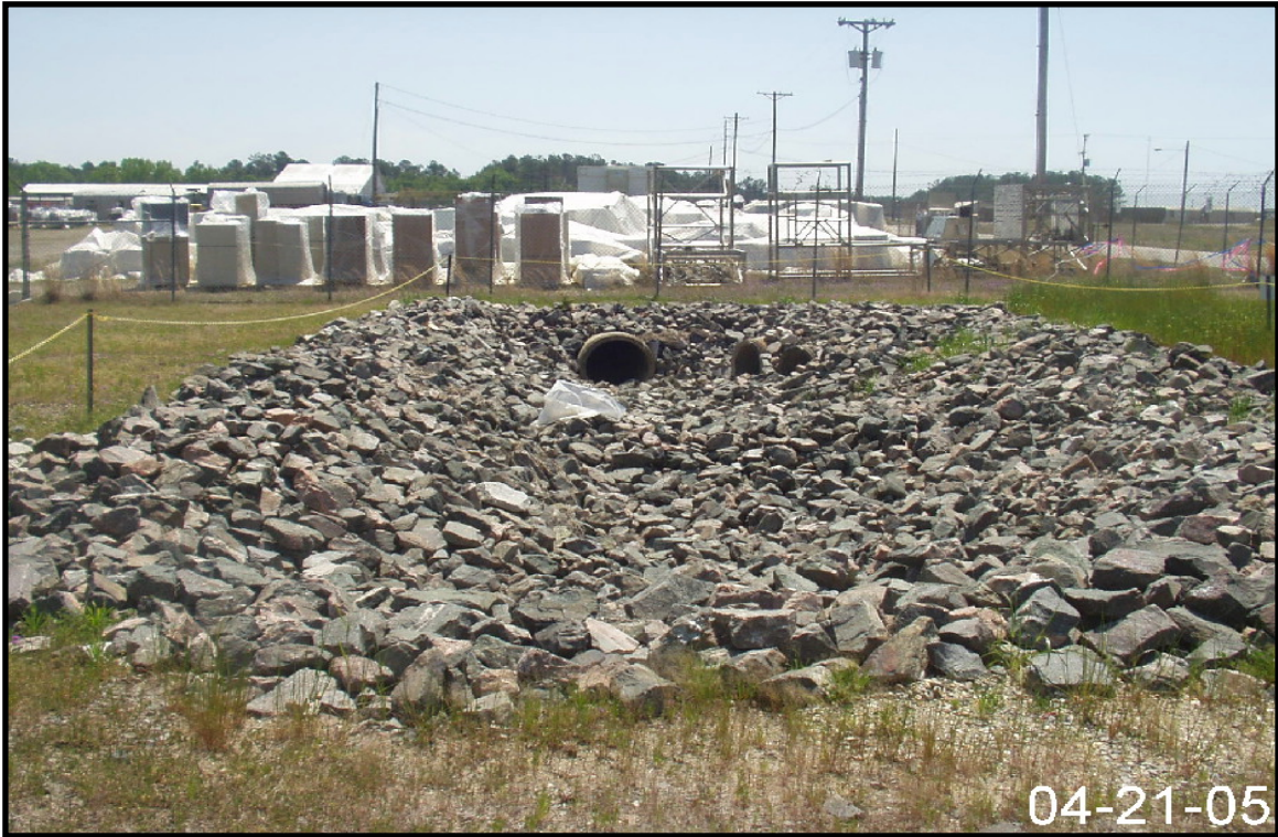
Figure 2-78. View of Storm Water Outfall N-2A.
