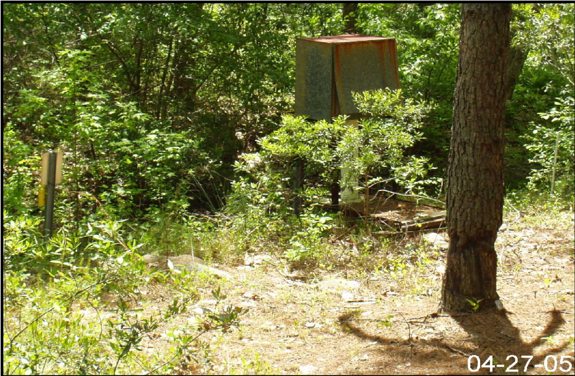
Figure 2-114. View of Storm Water Outfall P-13.
