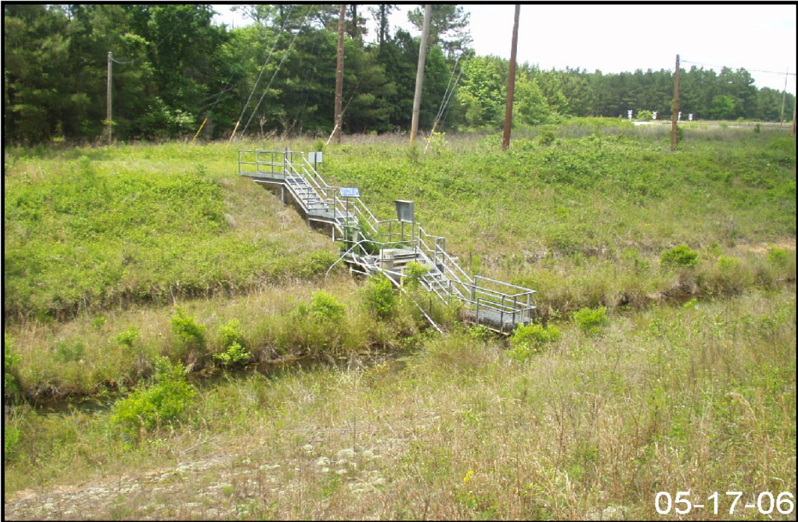
Figure 2-117. View of Storm Water Outfall P-19.
