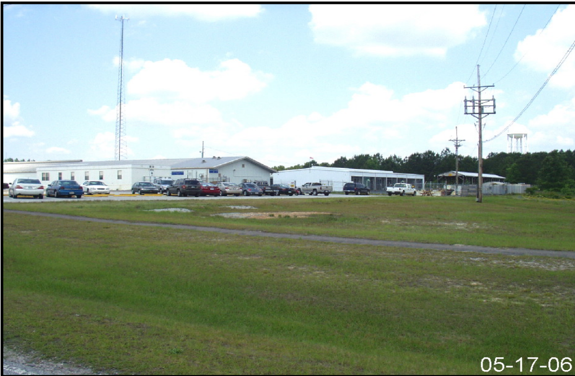
Figure 2-106. Representative View of Drainage Area for Storm Water Outfall N-15.
