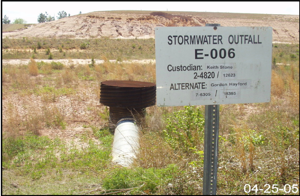
Figure 2-30. View of Storm Water Outfall E-06.
