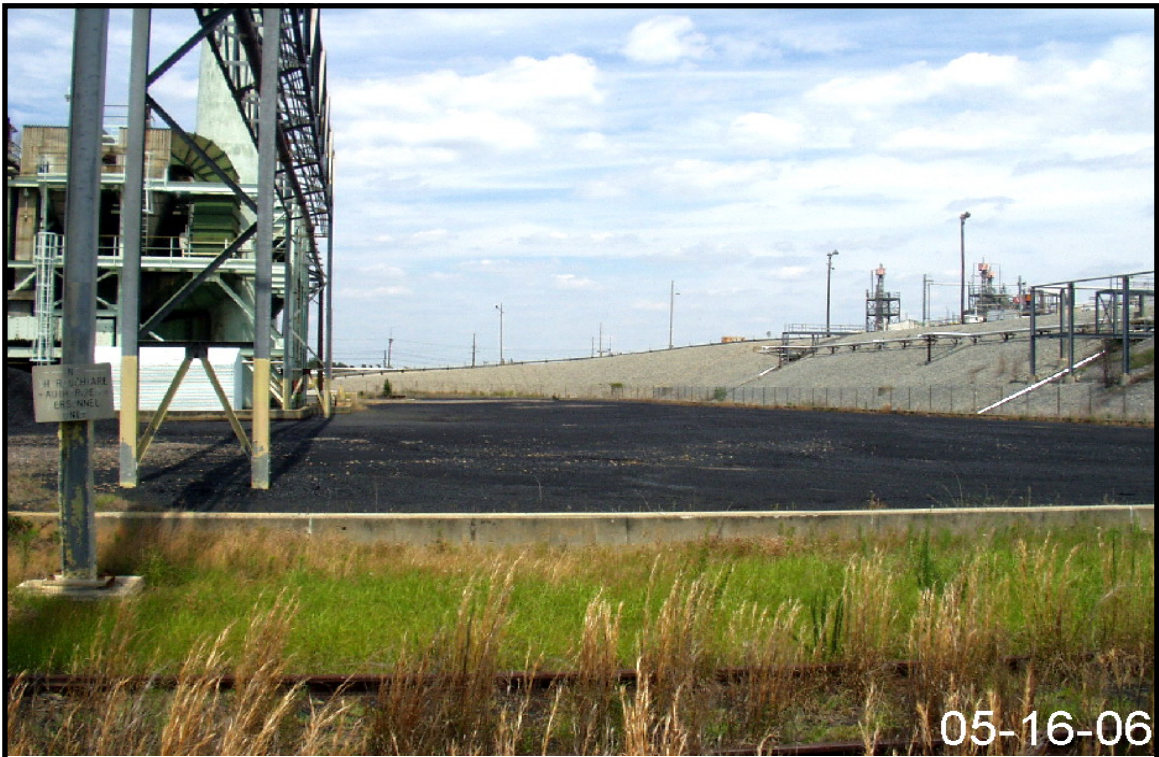
Figure 2-49. Representative View of Drainage Area for Storm Water Outfall H-7B.
