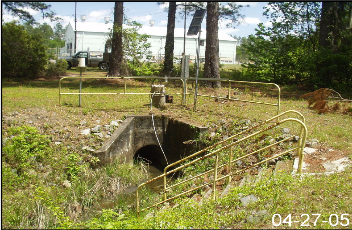
Figure 2-120. View of Storm Water Outfall Y-01.
