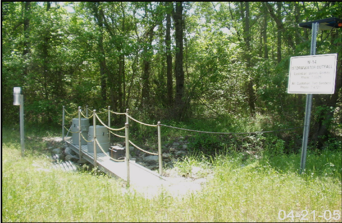
Figure 2-102. View of Storm Water Outfall N-14.
