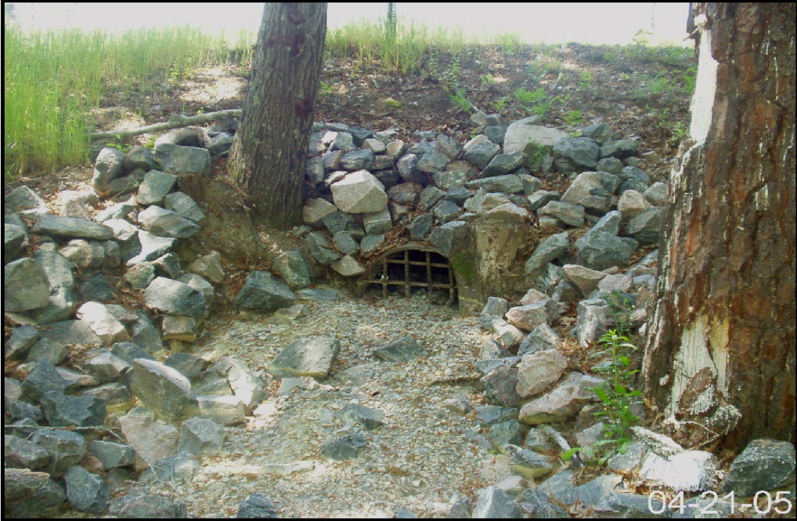
Figure 2-84. View of Storm Water Outfall N-05.
