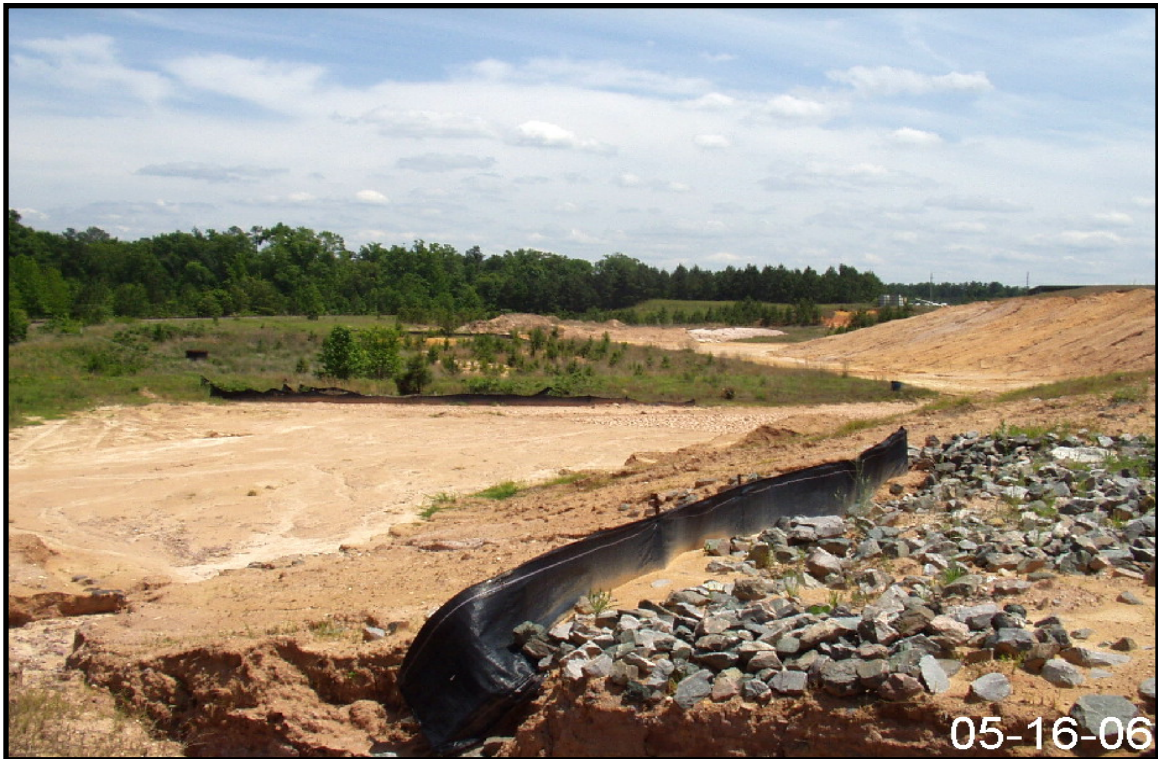
Figure 2-31. Representative View of Drainage Area for Storm Water Outfall E-06.
