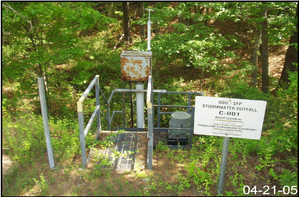
Figure 2-9. View of Storm Water Outfall C-01.
