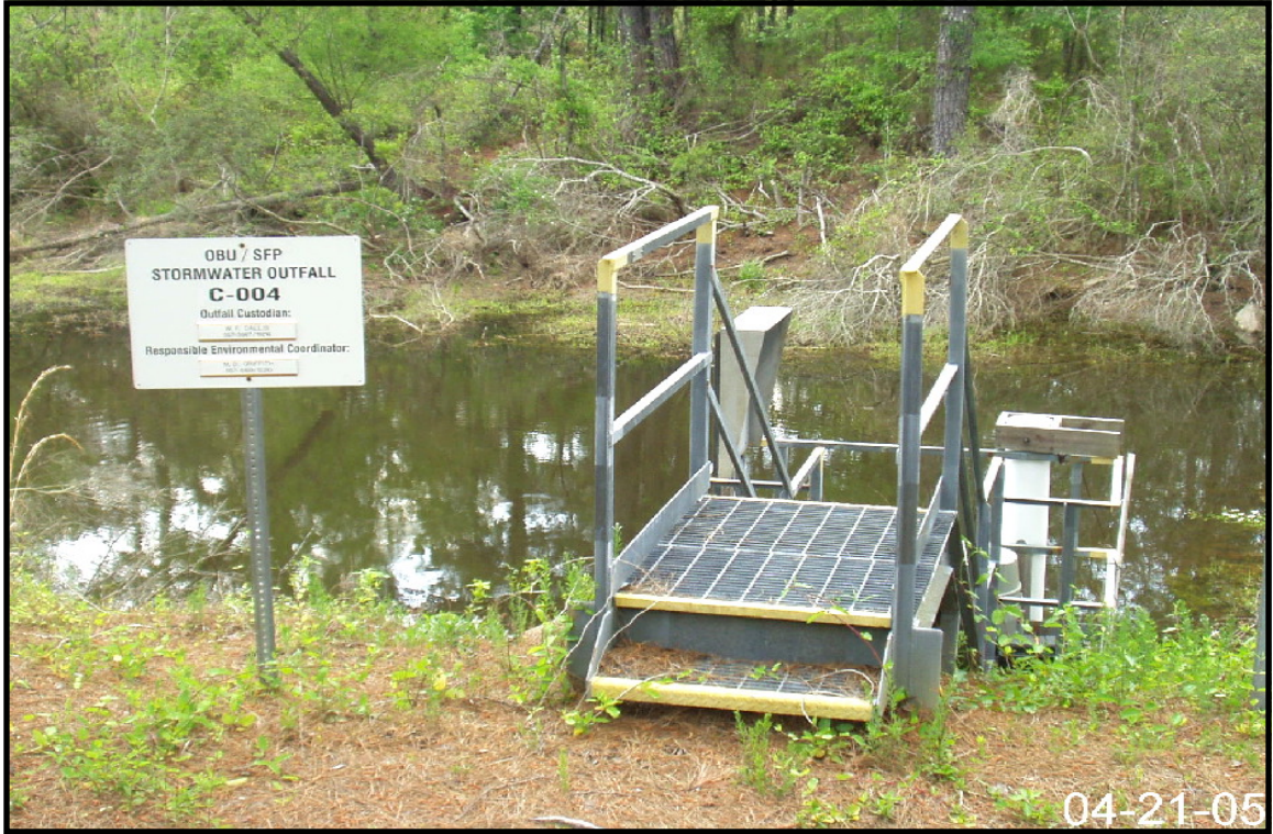
Figure 2-12. View of Storm Water Outfall C-04.
