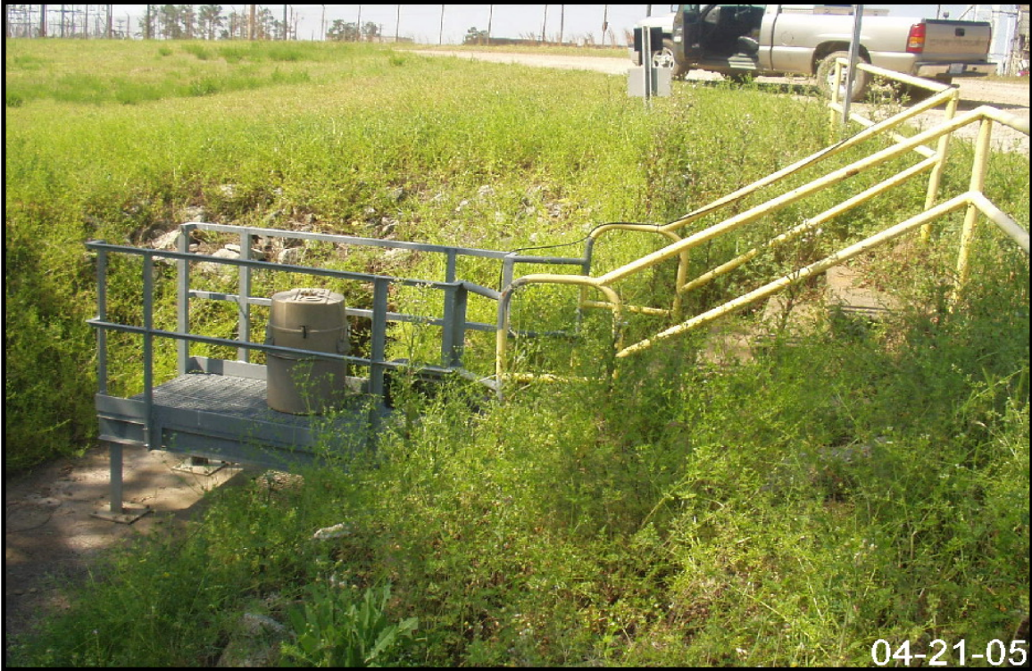
Figure 2-3. View of Storm Water Outfall A-08.
