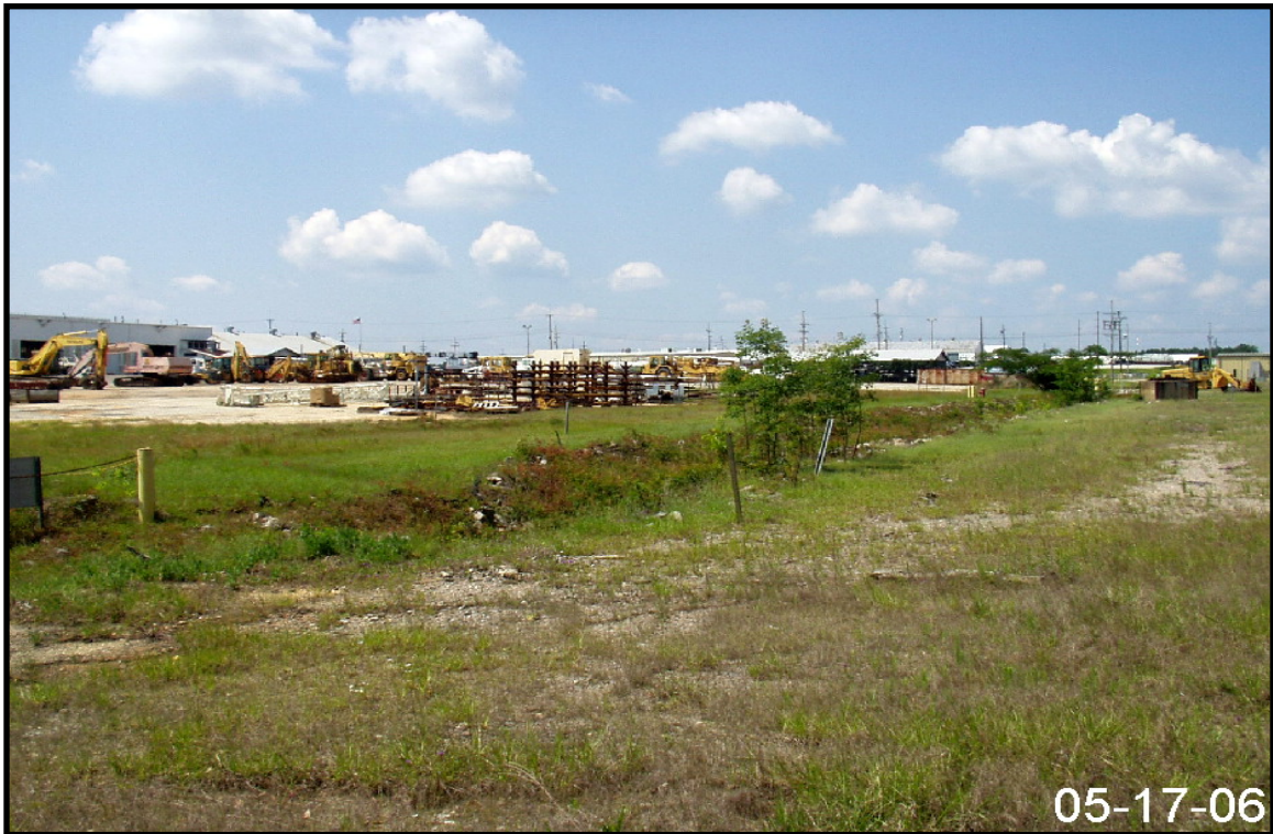
Figure 2-72. Representative View of Drainage Area for Storm Water Outfall N-01.
