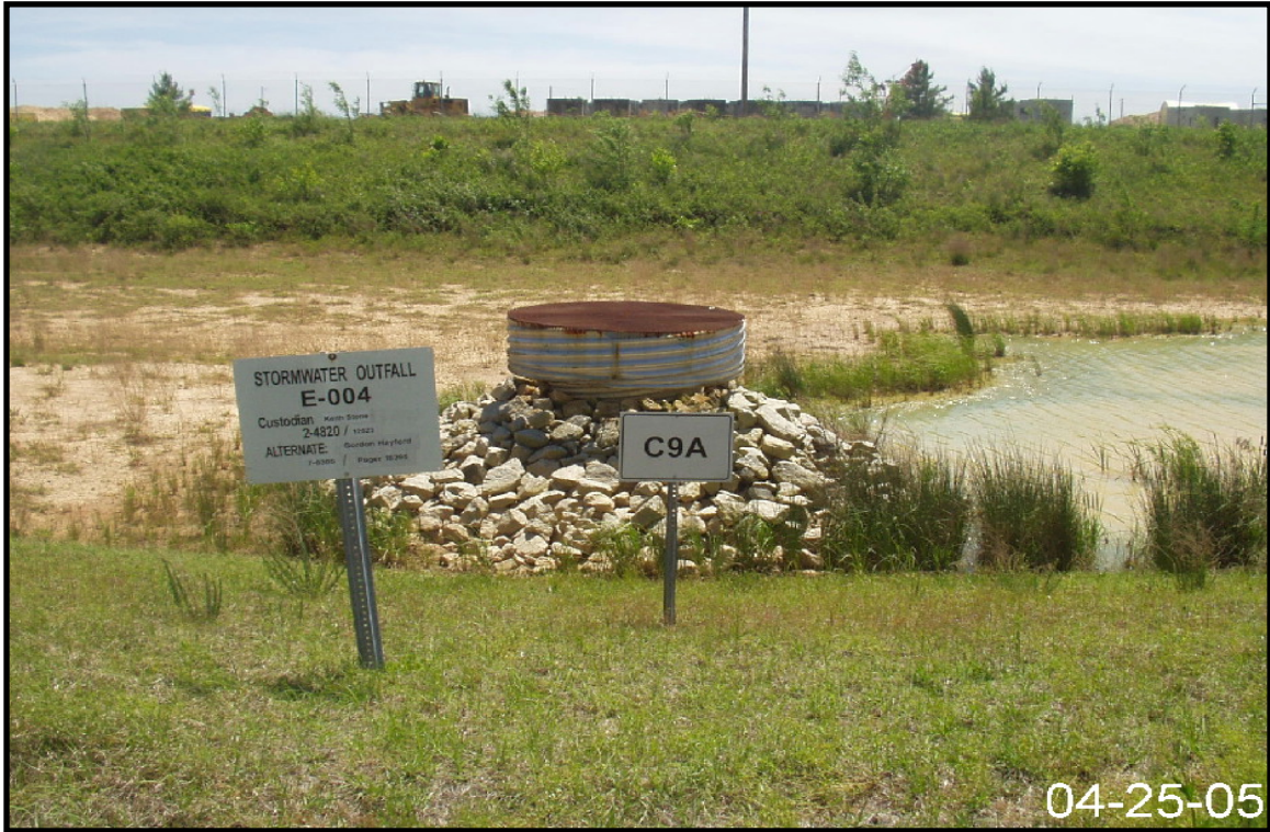
Figure 2-24. View of Storm Water Outfall E-04.
