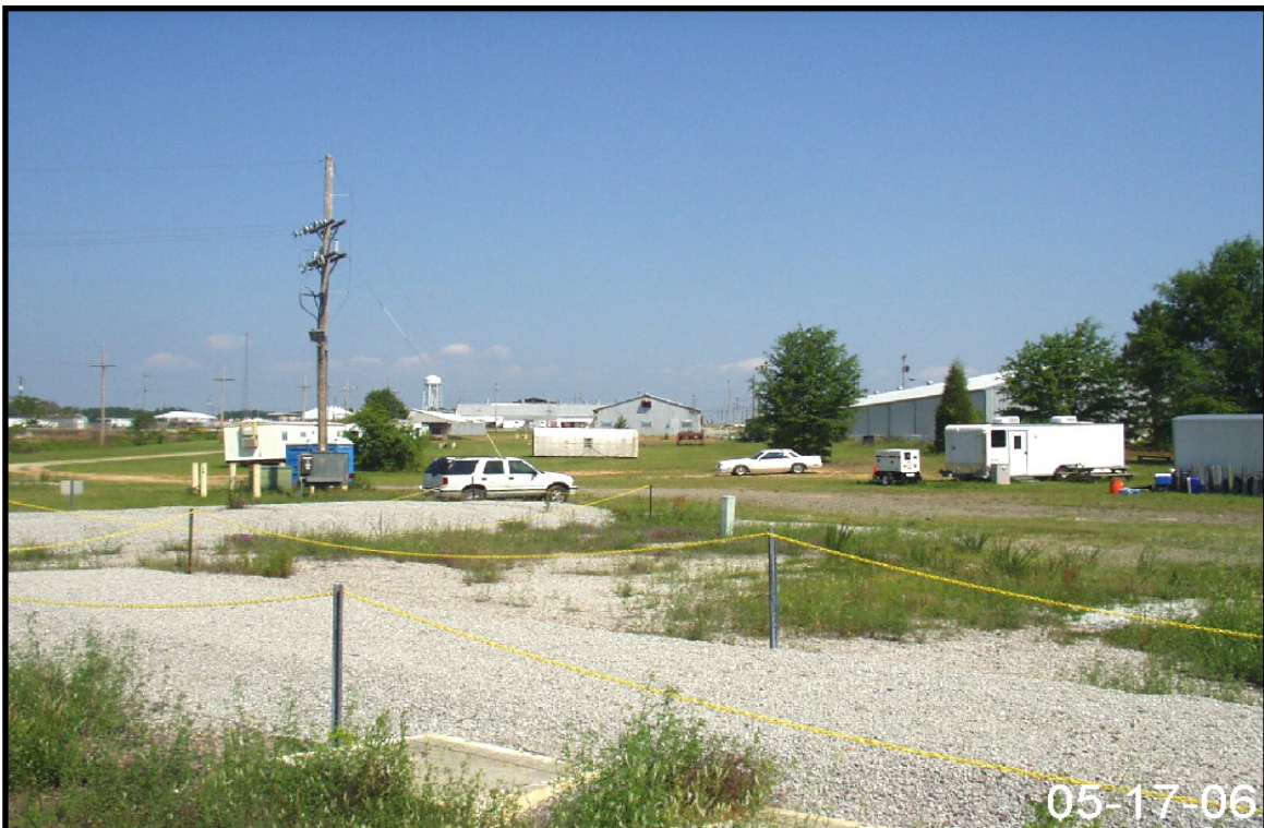
Figure 2-94. Representative View of Drainage Area for Storm Water Outfall N-12.
