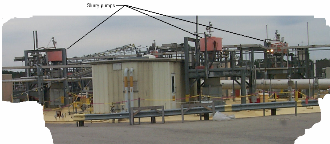
Figure 1: Typical Mixing or Slurry Pumps Installed on the Top of an Underground Tank at Savannah River Site
