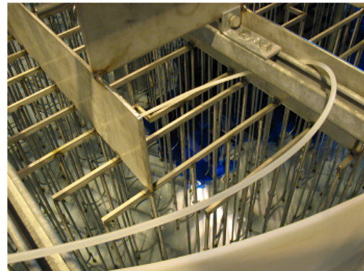
Dye Spreading Across the Tank Floor, B3 Riser, Near the Pump
