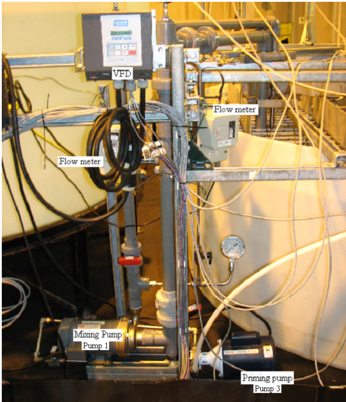
Figure 8: Mixing Pump for Pilot Scale Blending Tank
