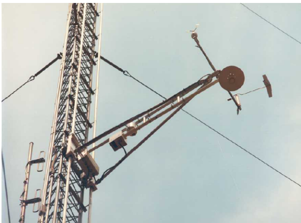
Fig. 3 Typical 62 m (200 ft) Rohn tower with instrument platform being raised by an electrically driven elevator.
