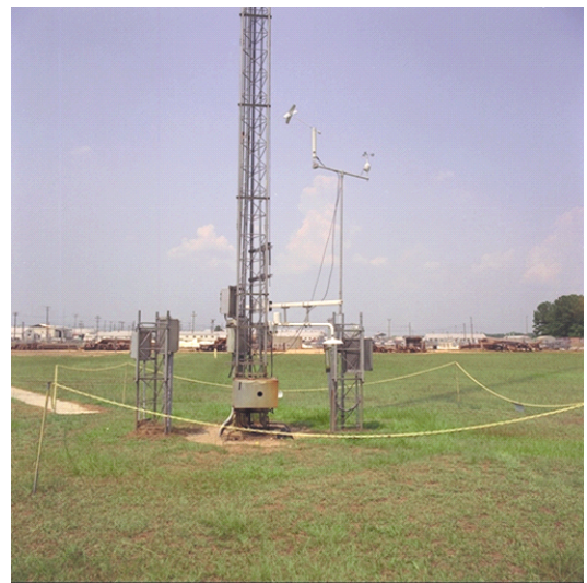
Fig. 6 The tower at the Climatology Facility tower with instrumentation at 4 levels to 62 m.
