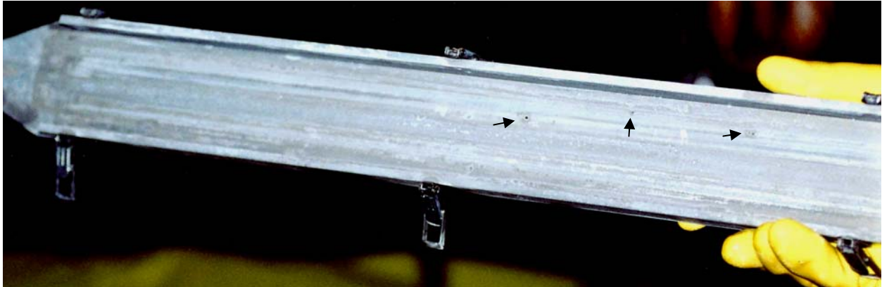
Figure 11. Pit locations are shown on interior surface of one clamping plate from B-3 fuel assembly in 2004. The pits appear to be in locations where fuel plates touch the clamping plate.
